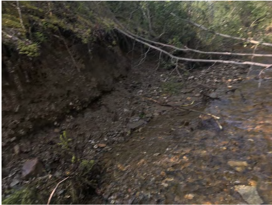
Photo 13 Adams Creek, KL_BO_AD03 (YPS-624) looking upstream.
