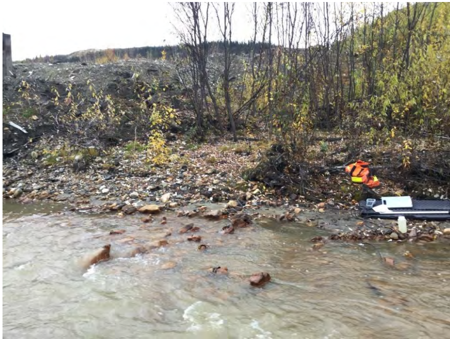
Photo 109 Hunker Creek, YPS-051, left bank.
