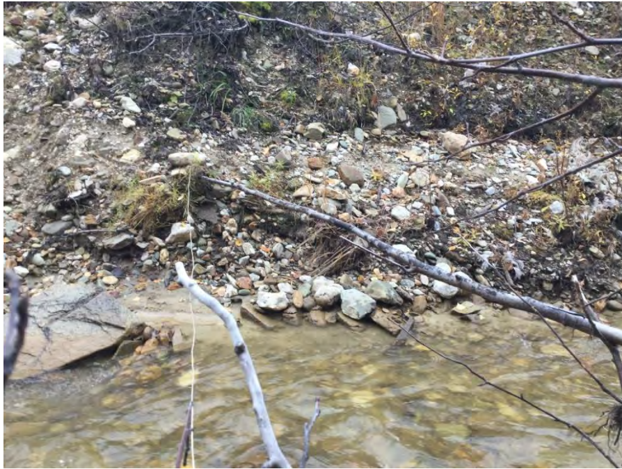
Photo 9 Adams Creek, KL_BO_AD02 (YPS-623) right bank.
