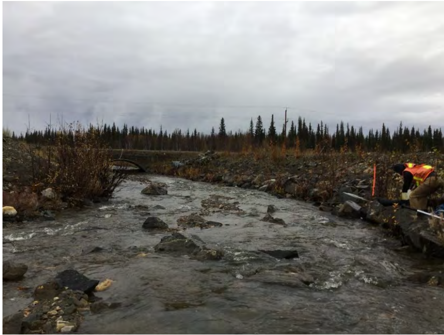
Photo 39 All Gold Creek, KL_AL01 looking downstream.
