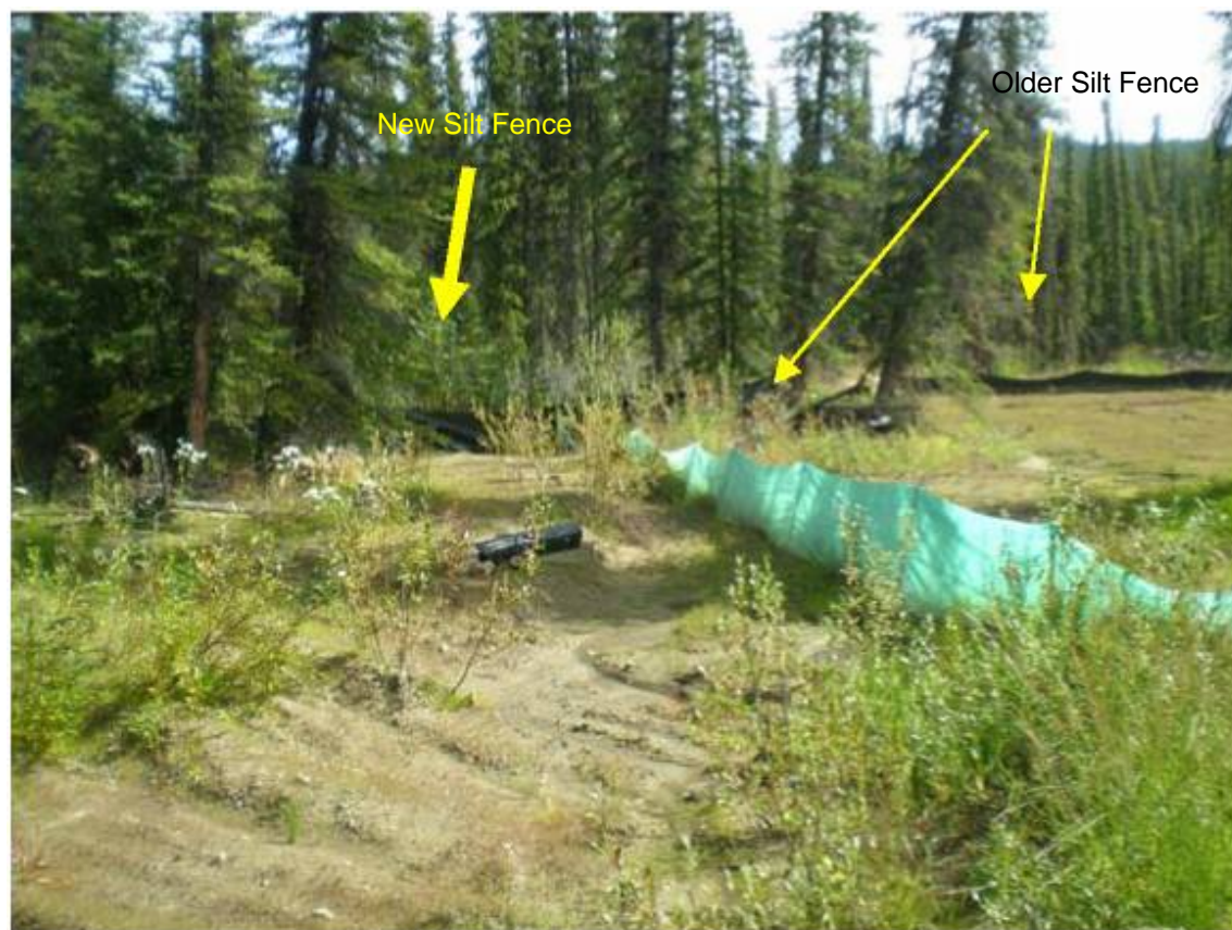
Photograph 8: An additional row of silt fencing was added beyond the green silt fence on August 5 to control further sediment movement towards Williams Creek.
