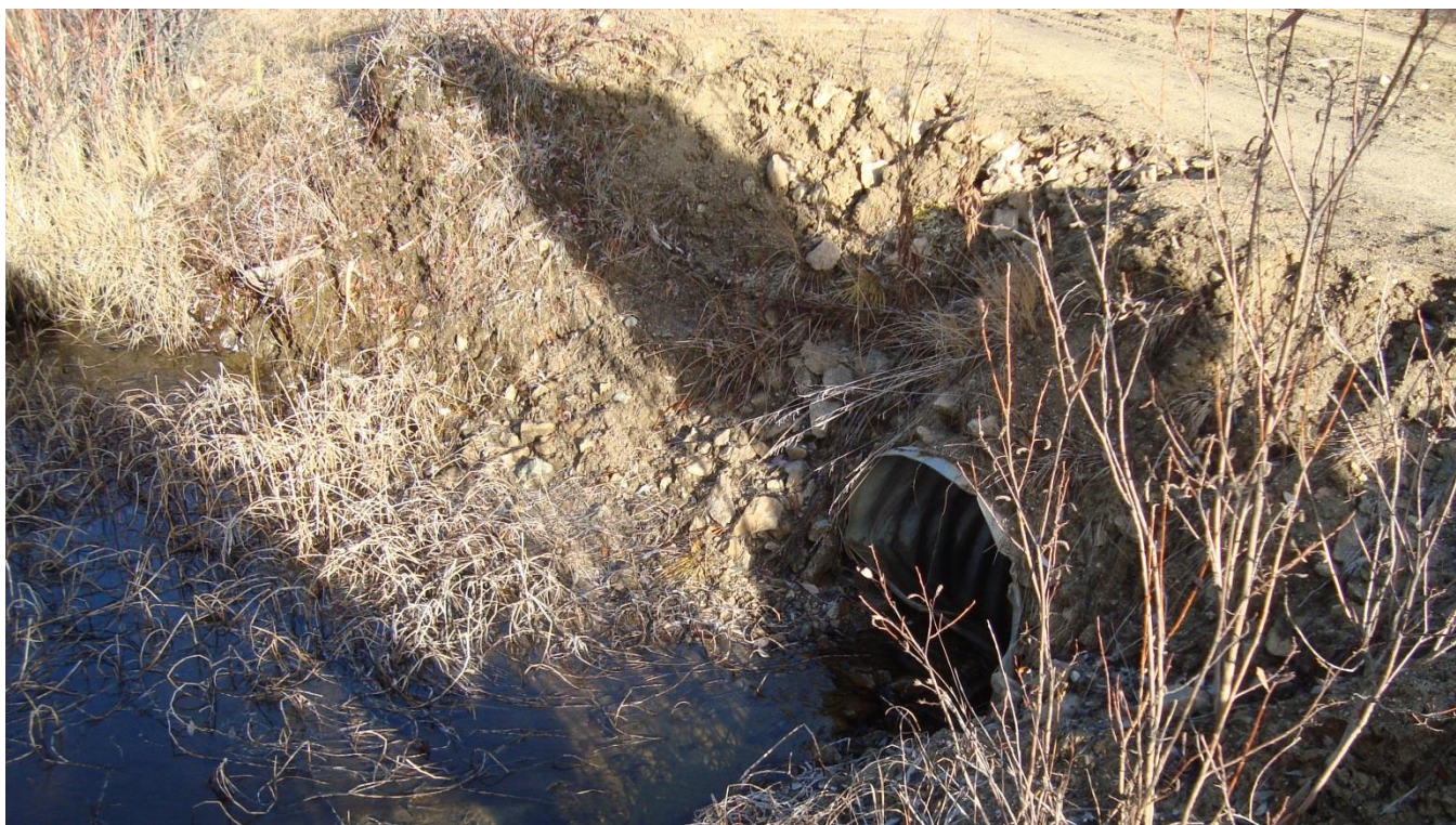
Photograph 16: View looking east of erosion above culvert on access road at North Williams Creek
