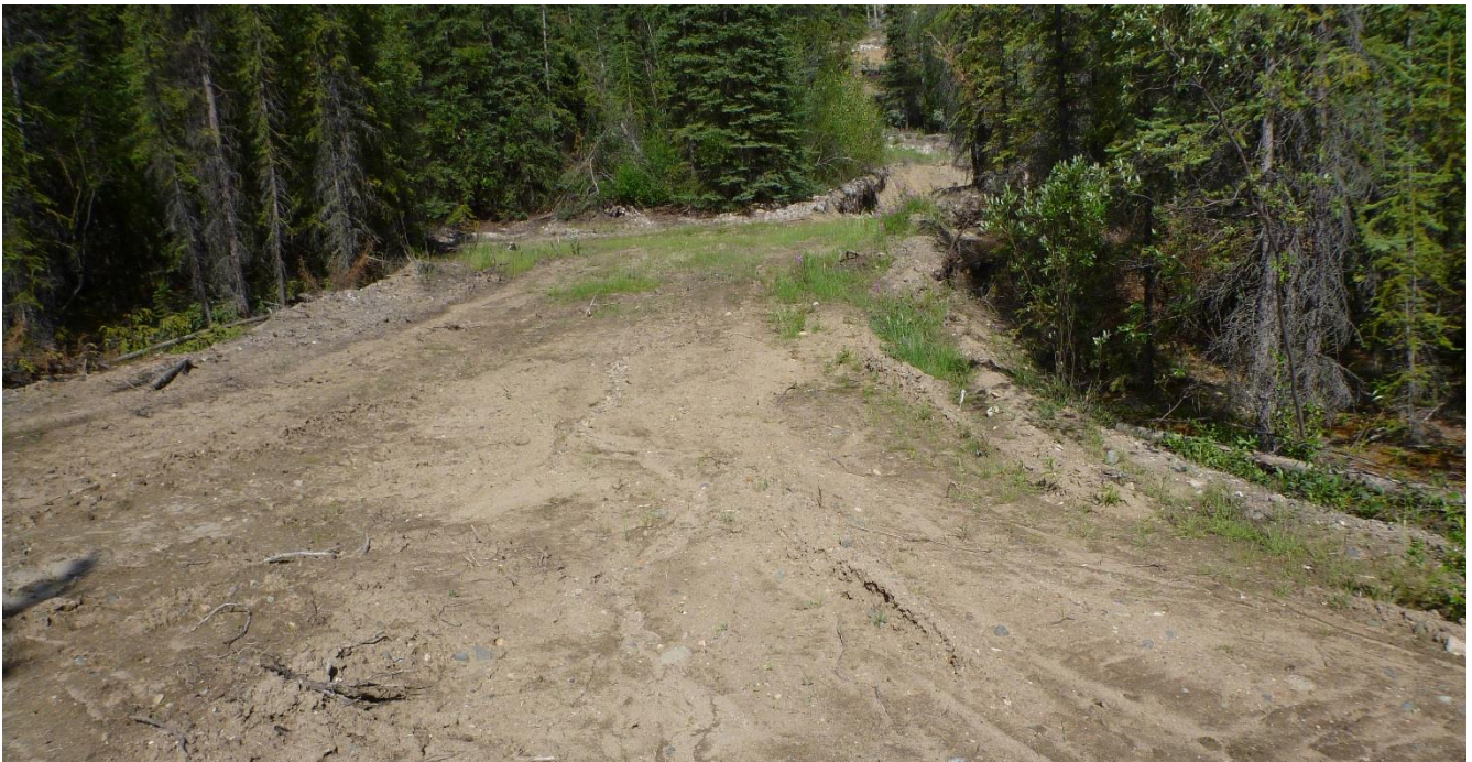
Photograph 10: Erosion of sediment from drill pad and access road
