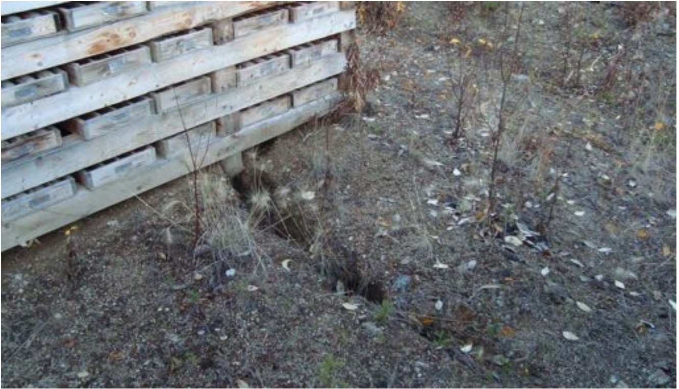
Photograph 1: Crack beneath core storage rack
