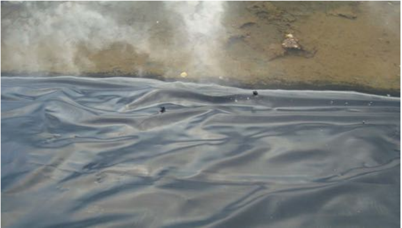
Photograph 13: Liner damage at fuel storage area
