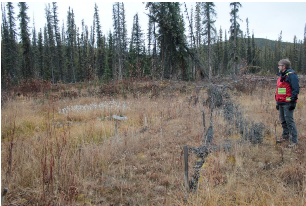
Photograph 8: Vegetation growth around sediment fencing
