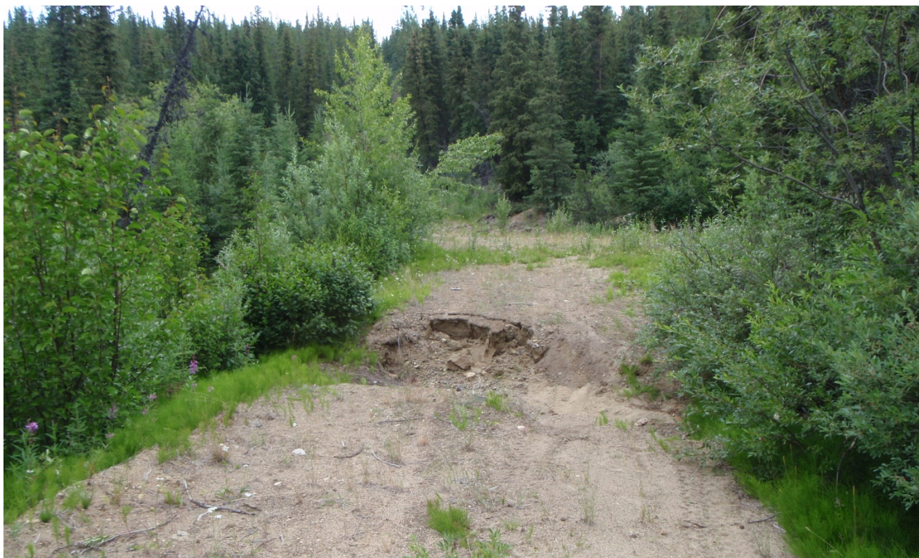
Photograph 20: Erosion on road near North Williams Creek crossing.
