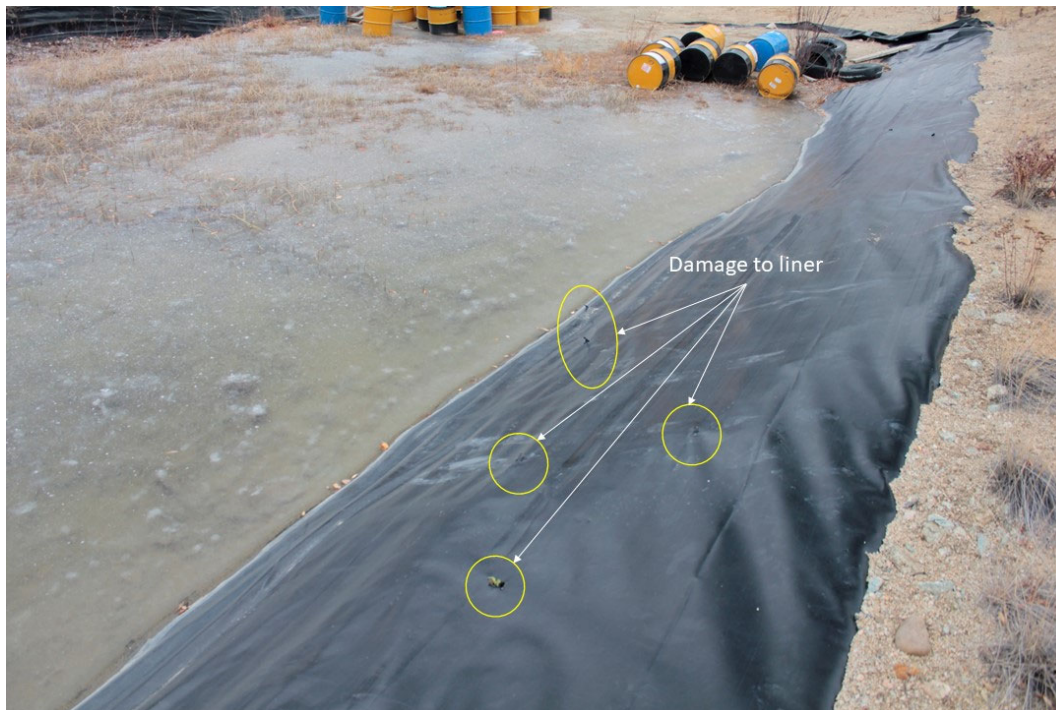
Photograph 11: Liner damage at fuel storage area
