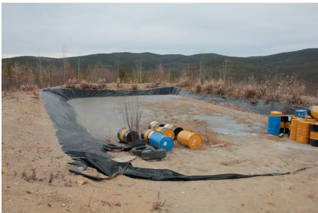
Photograph 10: Lined basin at fuel storage area
