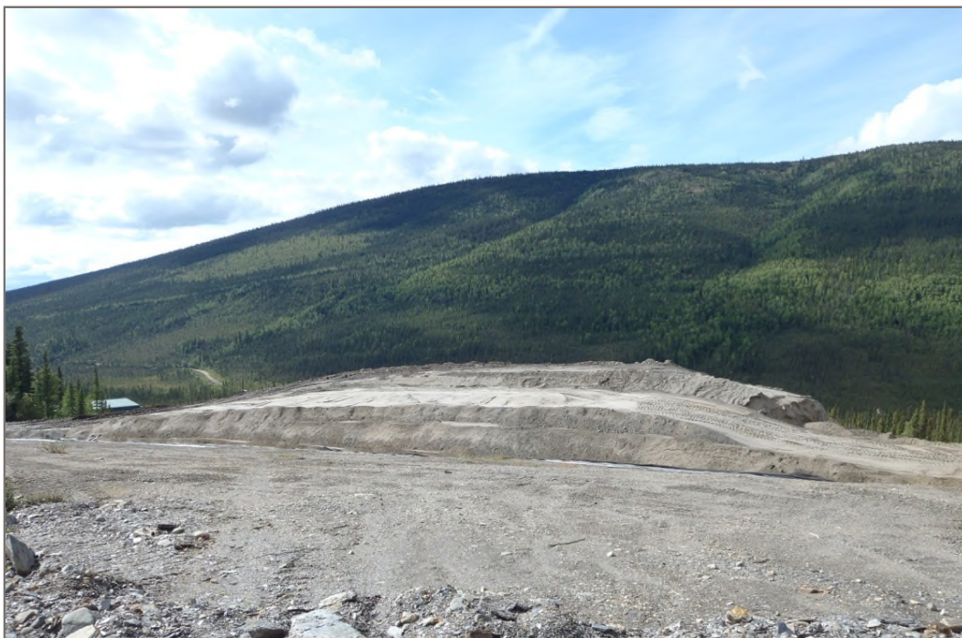
Photo 24: Dry Stacked Tailings Facility Top of facility where tailings placement will continue Facing west – August 13, 2014
