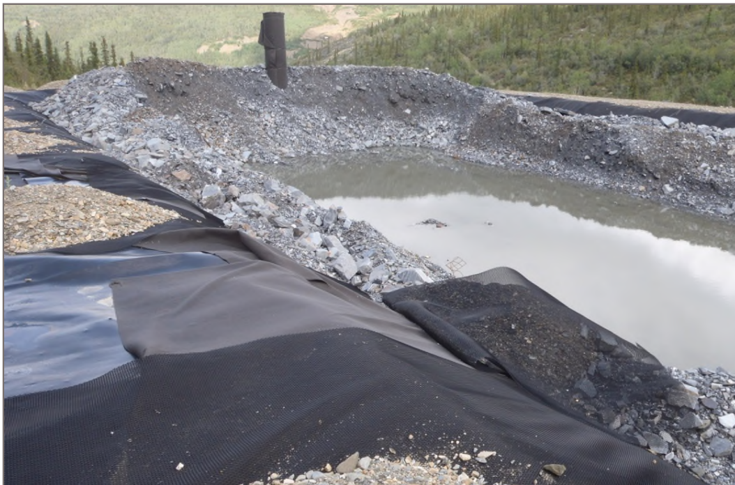
Photo 4: PAG Waste Storage Facility Liner components displaced due to wind Facing east – August 12, 2014
