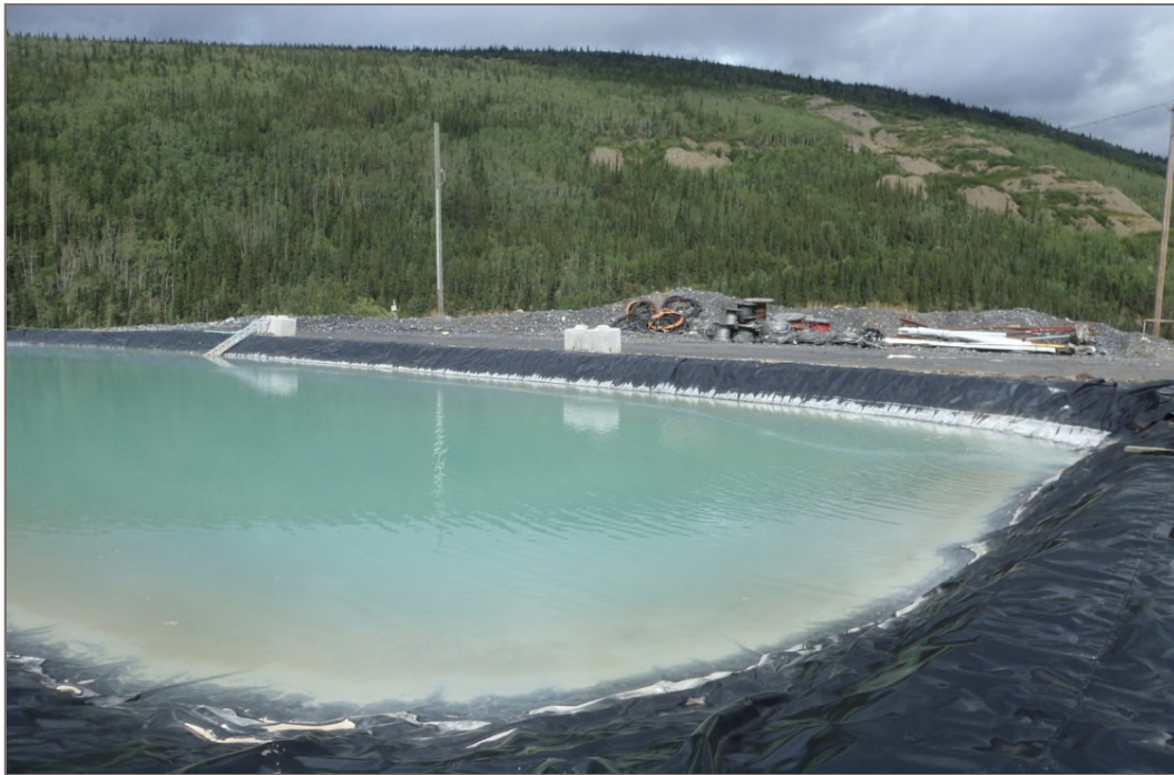
Photo 7: Bellekeno 625 Water Treatment Ponds Intact perimeter berms and liners Facing east – August 12, 2014
