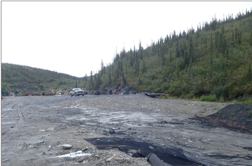
Photo 3: PAG Waste Storage Facility Laydown area graded toward facility entrance Facing south – August 12, 2014
