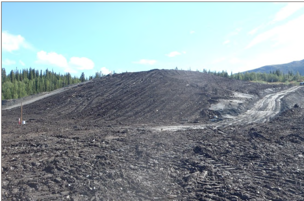
Photo 23: Dry Stacked Tailings Facility Progressive reclamation of upper bench (cover and seed mixture applied) Facing east – August 13, 2014
