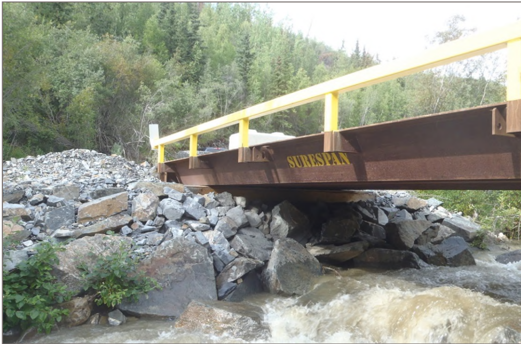
Photo 15: Lightning Creek Bridge Abutments (Onek Road) Rip-rap armouring bridge abutments Facing north – August 12, 2014
