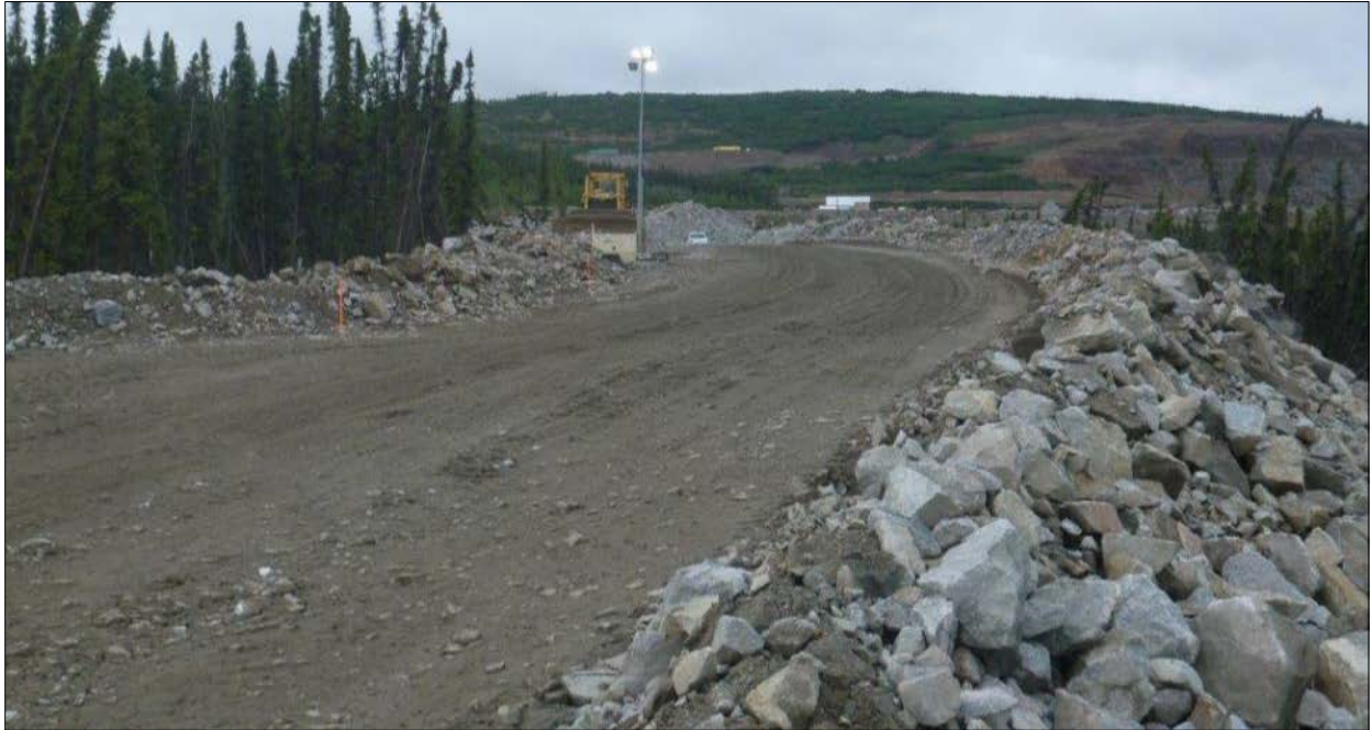
Picture 9-1: A view looking west of the segment C lined ditch embankment fill
