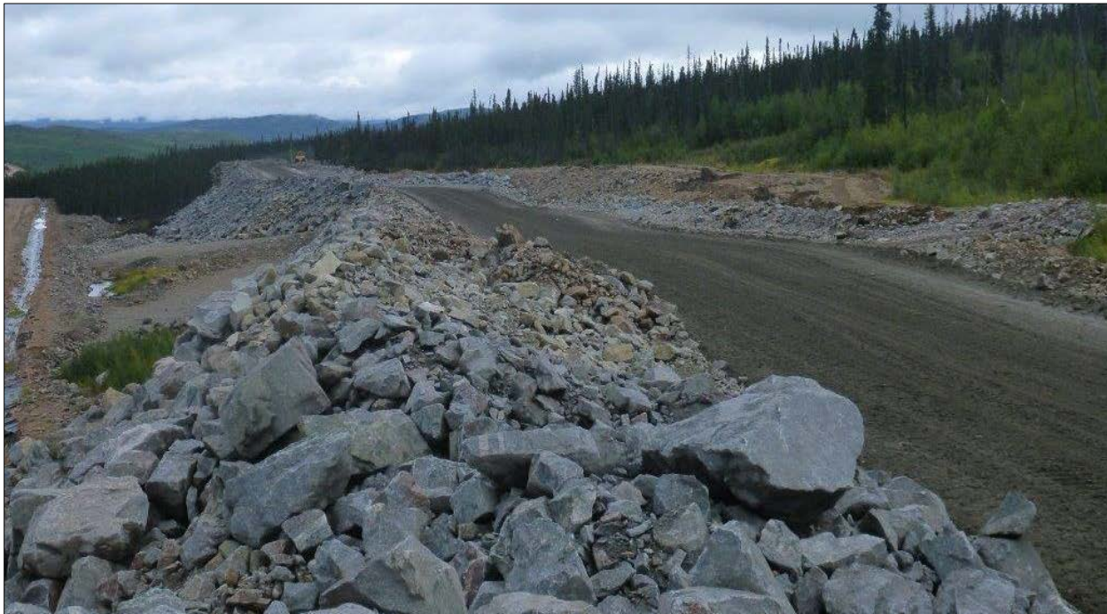
Picture 9-2: A view looking east of the segment A and B ditch and buttress
