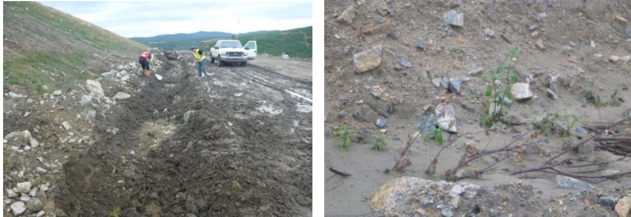
Picture 8-7: Planting willow on the MWD and the trench filled in after a rain storm
