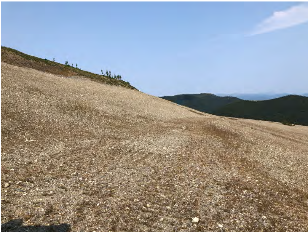
Photo 24: Regraded slopes of Jewelbox waste rock dump
