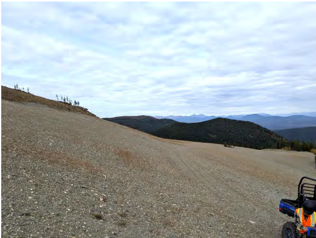
Photo 24: Regraded slopes of Jewelbox waste rock dump
