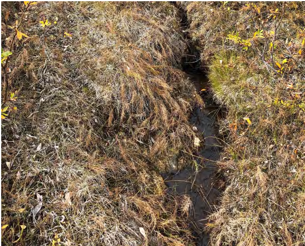
Photo 6: Seepage at toe of North Dam, mainly due to hillside springs
