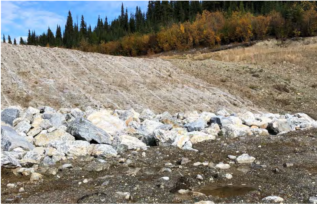
Photo 17: View of the rock protection along the downstream toe of the SRS on east side
