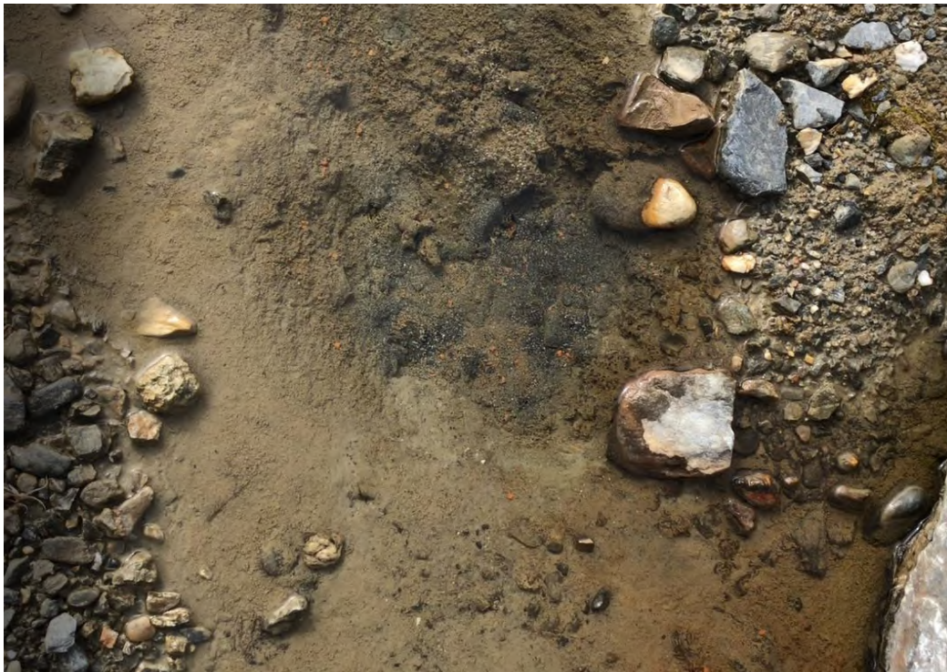
Photo 18: small boils at toe of SRS. Due mainly to local spring activity.
