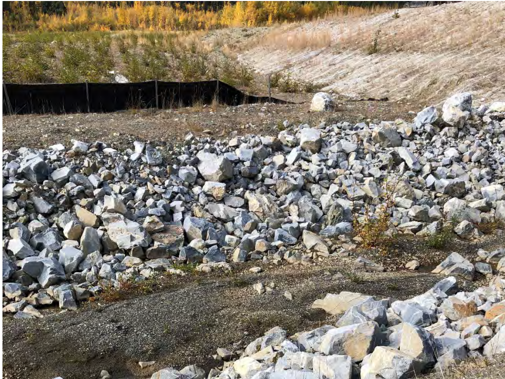
Photo 16: Plunge pool below SRS spillway
