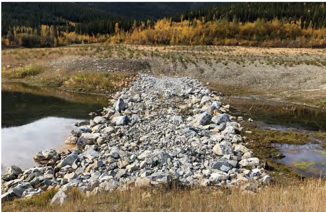
Photo 14: Rock Cofferdam above SRS looking west
