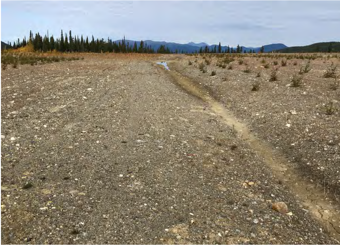
Photo 9: View looking north of drainage swale on tailings till cover
