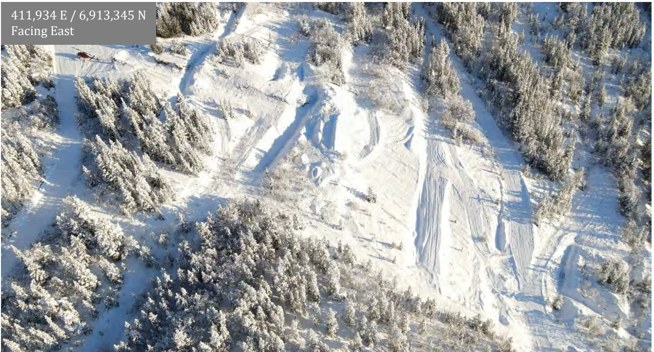
Photo 8: Site access roads at the southern point of the proposed open pit
