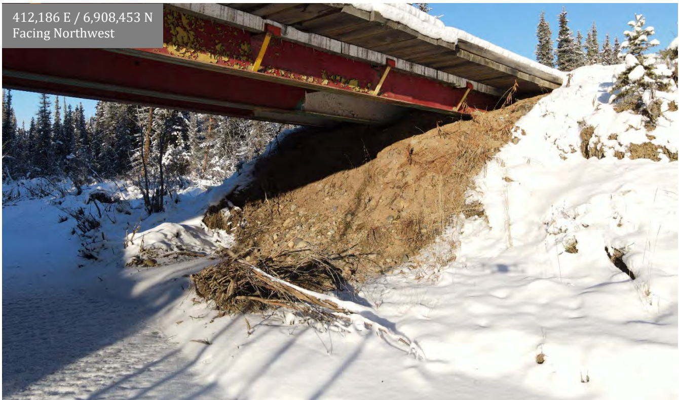
Photo 13: Merrice Creek bridge north abutment
