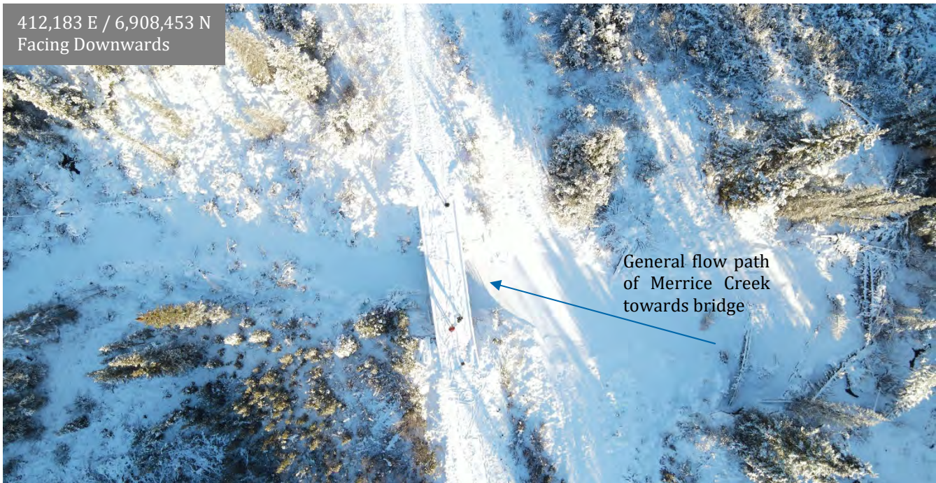
Photo 15: Aerial view of Merrice Creek bridge
