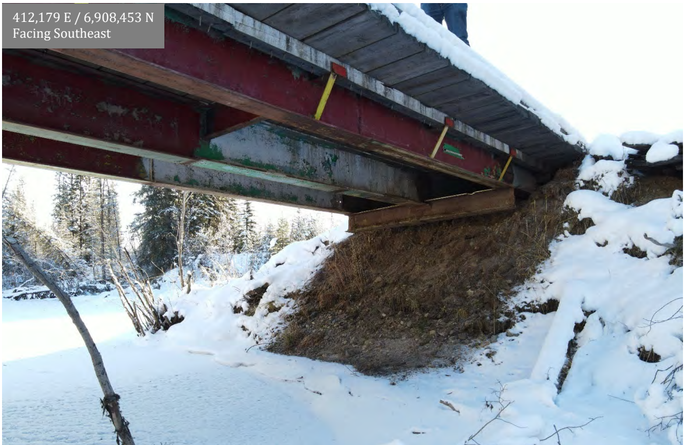
Photo 14: Merrice Creek bridge south abutment
