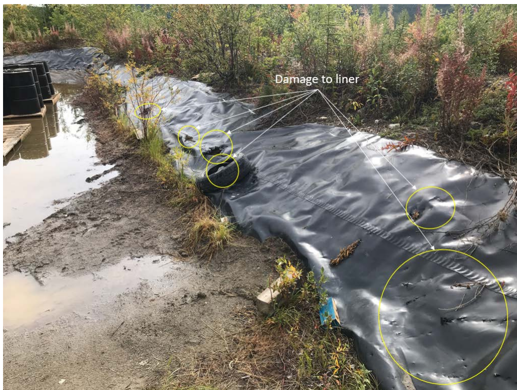
Photograph 7: Liner Damage along South Slope at Fuel Storage Area Looking East
