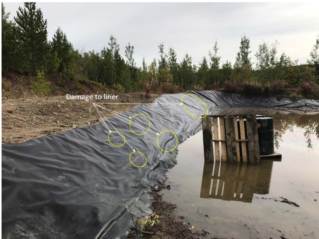
Photograph 6: Liner Damage along North Slope at Fuel Storage Area Looking East
