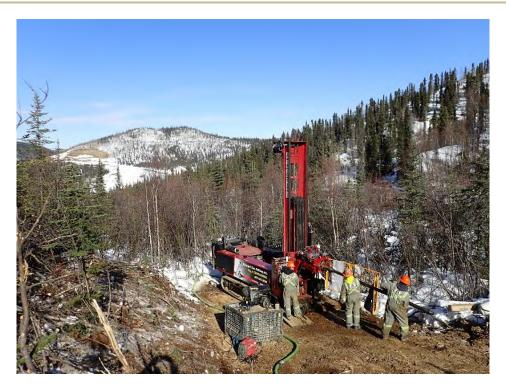
Photo 1: Compact crawler TerraSonic CC150 Drill Rig, Borehole GT18-05 site. Eagle Pup WRSA, looking north. Photo taken April 9, 2018
