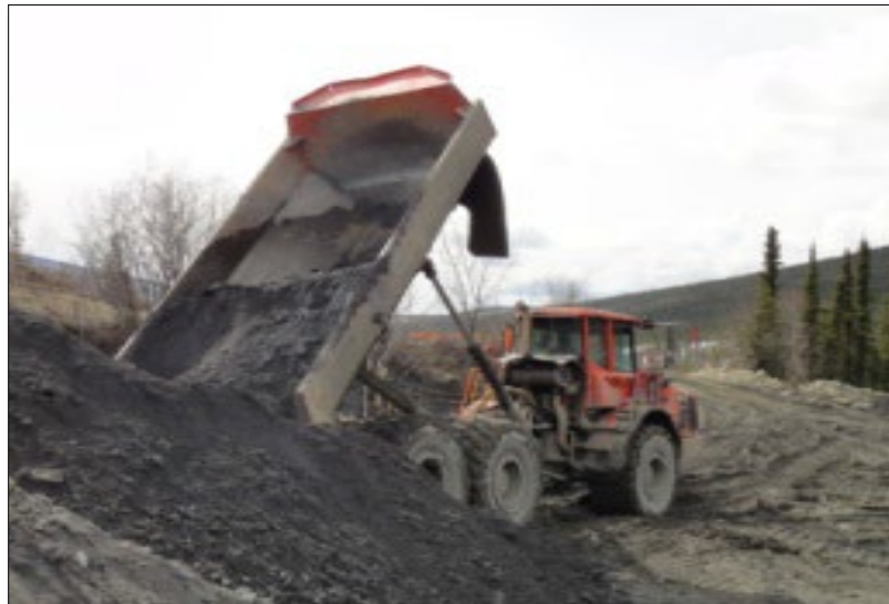
Photo 4-1: Run of Mine (ROM) Coarse Ore Storage
