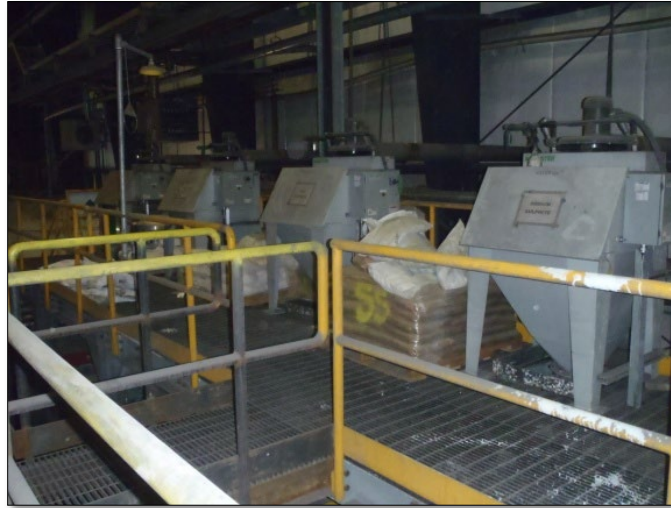
Photo 7-6: Reagent Mixing Station
