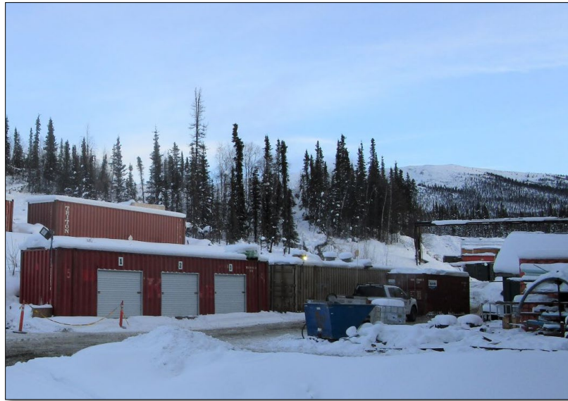
Photo 3-5: Mill Cold Storage
