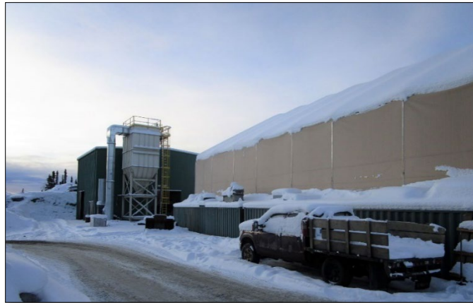
Photo 3-2: Crusher building, baghouse, fine ore storage tent and cold storage containers
