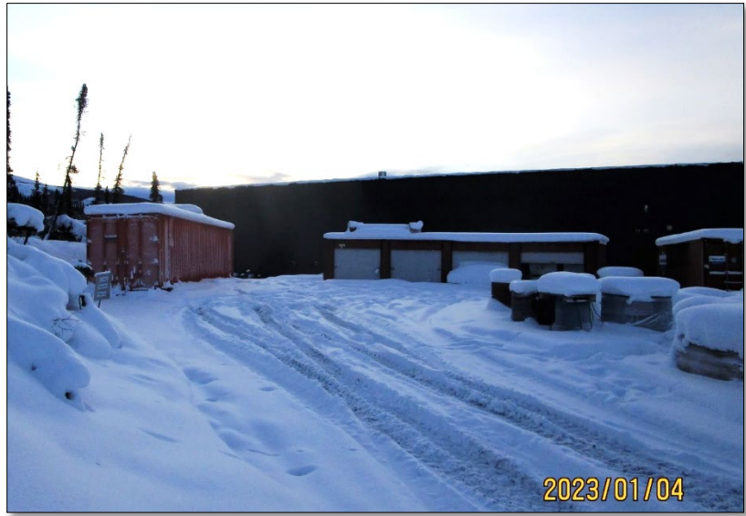
Photo 7-7: Reagent Laydown Yard
