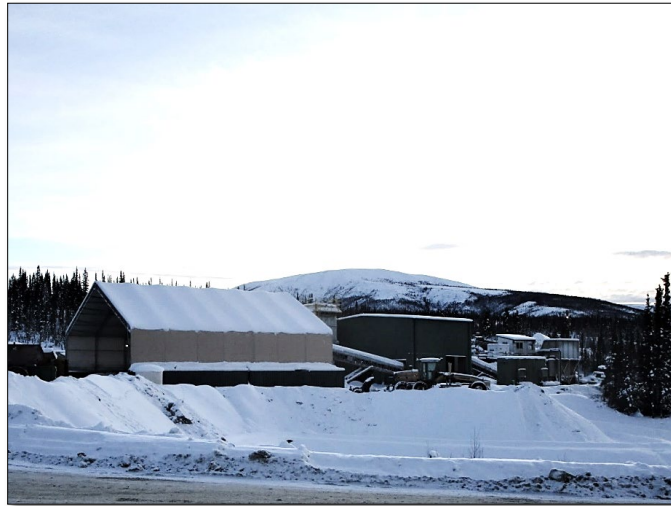
Photo 7-1: Fine Ore Storage, Secondary and Primary Crusher Building
