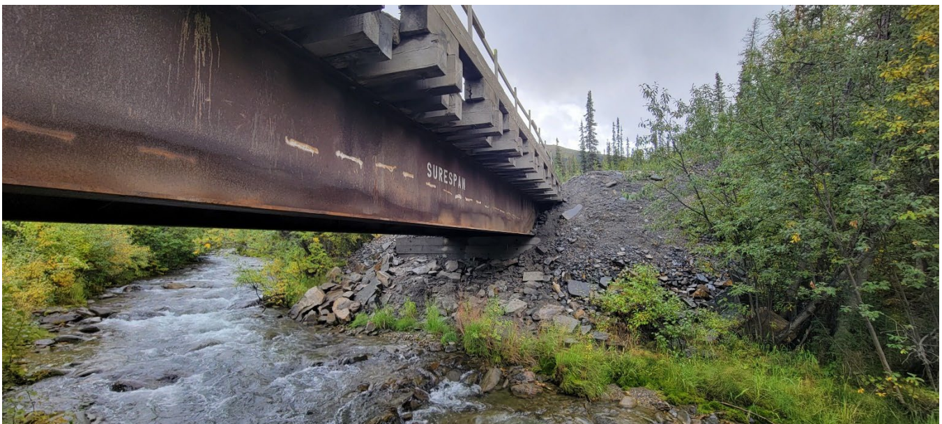
Photo 6: Lightning Creek Bridge - Bellekeno Haul Road, abutment armoring (I. MacIntyre, Aug. 28, 2022)
