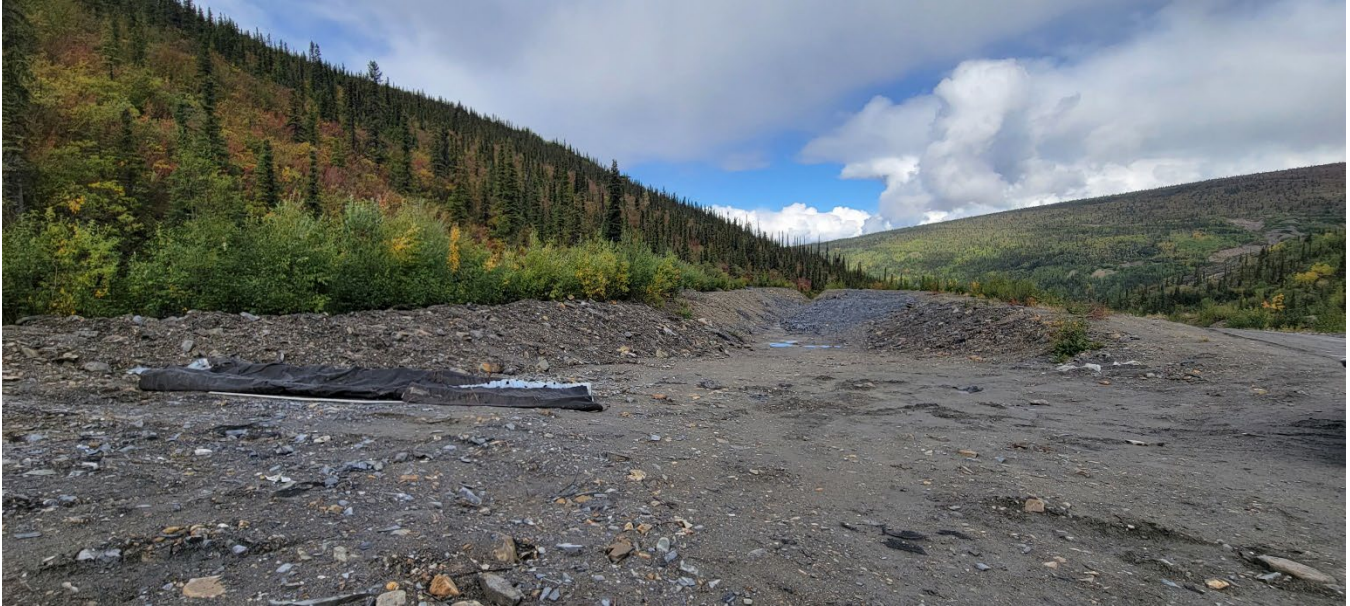
Photo 1: Bellekeno PAG Storage Facility, facing north (I. MacIntyre, Aug. 28, 2022)
