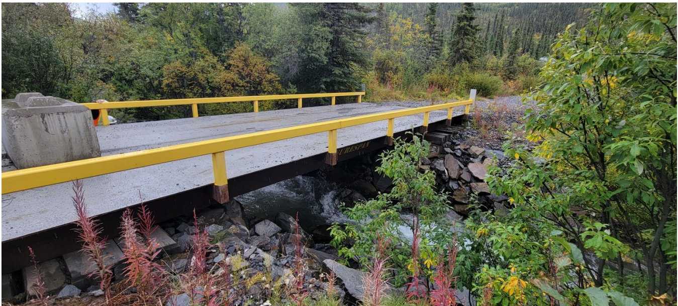
Photo 8: Lightning Creek Bridge - Onek Road (I. MacIntyre, Aug. 28, 2022)
