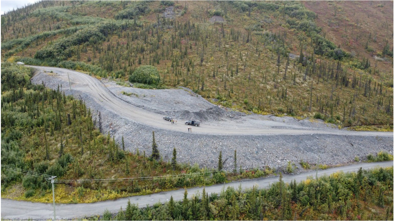
Photo 2: Bellekeno Road Waste Rock Pile, facing southwest (I. MacIntyre, Aug. 28, 2022)
