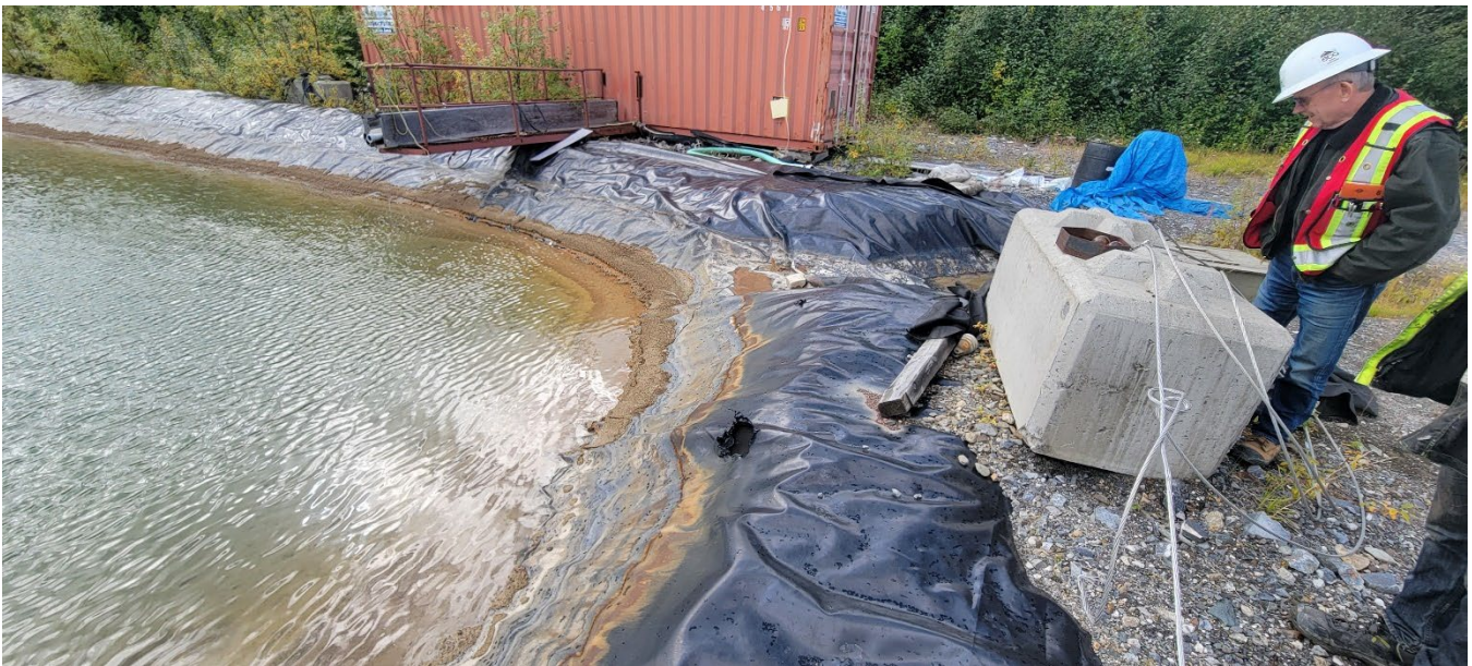
Photo 4: Bellekeno 625 Water Treatment Ponds, north end, rip visible (I. MacIntyre, Aug. 28, 2022)
