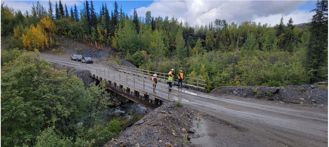
Photo 5: Lightning Creek Bridge - Bellekeno Haul Road (I. MacIntyre, Aug. 28, 2022)
