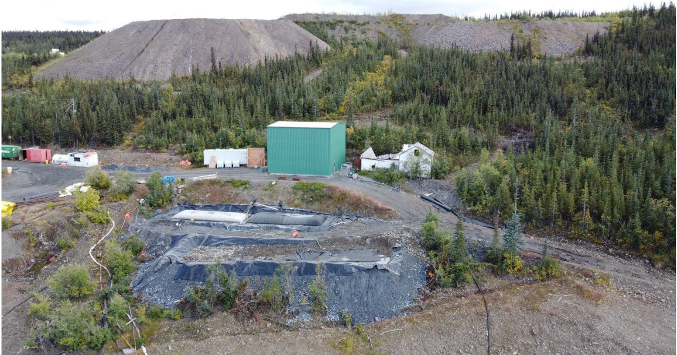
Photo 18: Birmingham Mine Sludge Waste Containment Facility – buried organics and trees visible in bottom of frame. (I. MacIntyre, Aug. 28, 2022)
