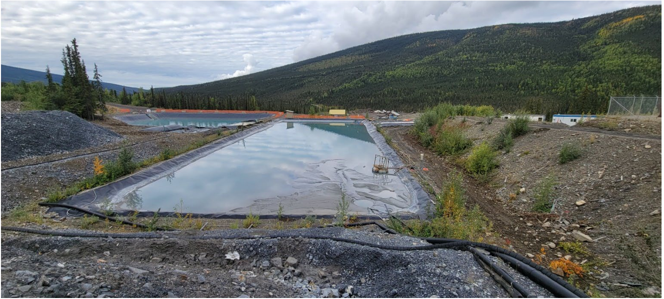
Photo 10: Mill water storage ponds – facing southwest (I. MacIntyre, Aug. 28, 2022)
