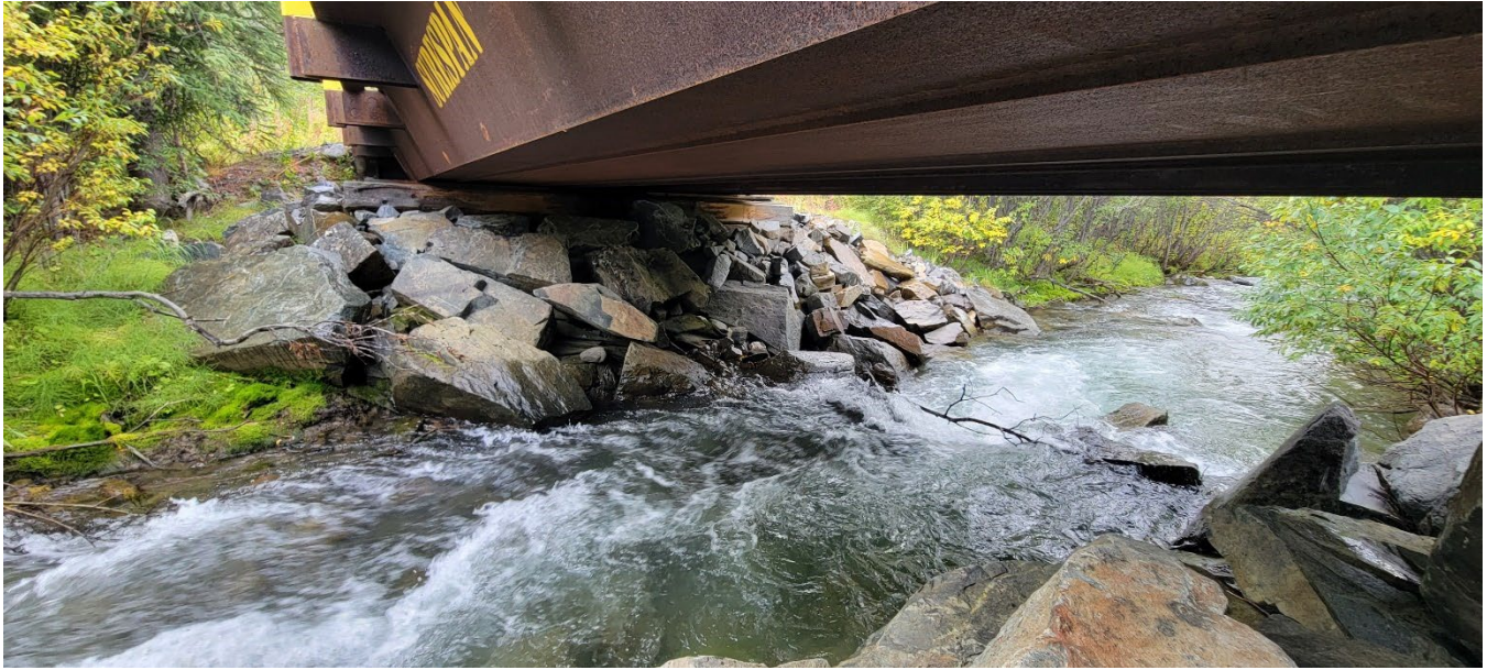
Photo 9: Lightning Creek Bridge – abutment riprap (I. MacIntyre, Aug. 28, 2022)
