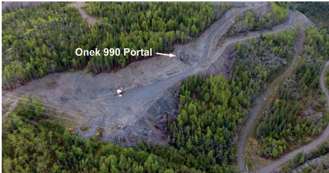
Figure 7-8 Onek Mine Surface Overview
