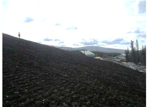
Photo 8: Covered DSTF mid-slope looking south
