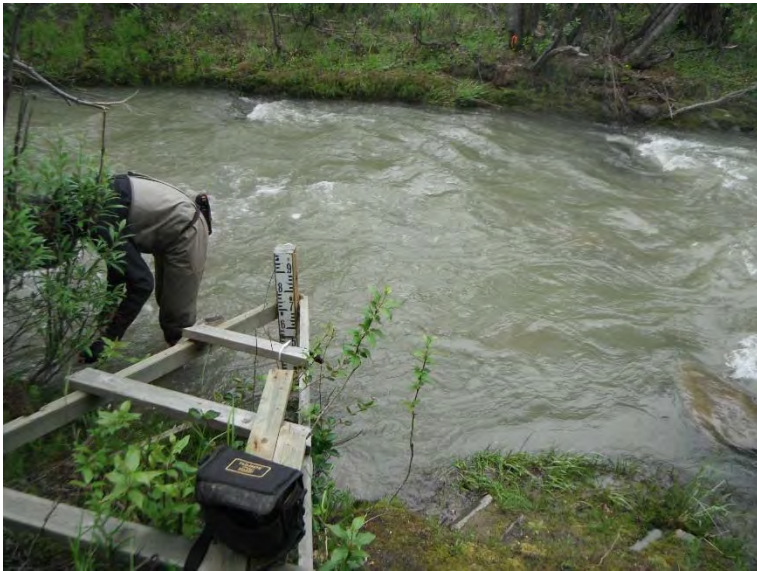
Photo 5: KV-41, staff gauge and aging wooden cribbing structure, June 16 th , 2016.
