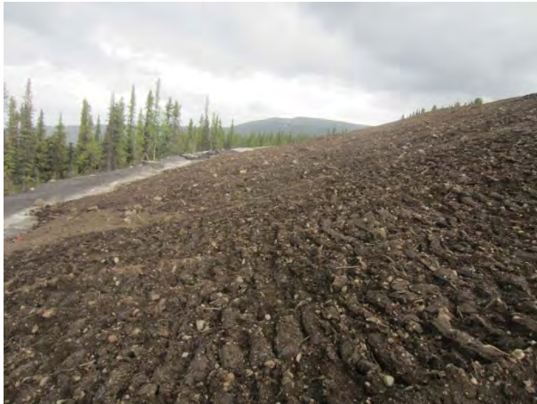
Photo 7: Covered DSTF toe looking north
