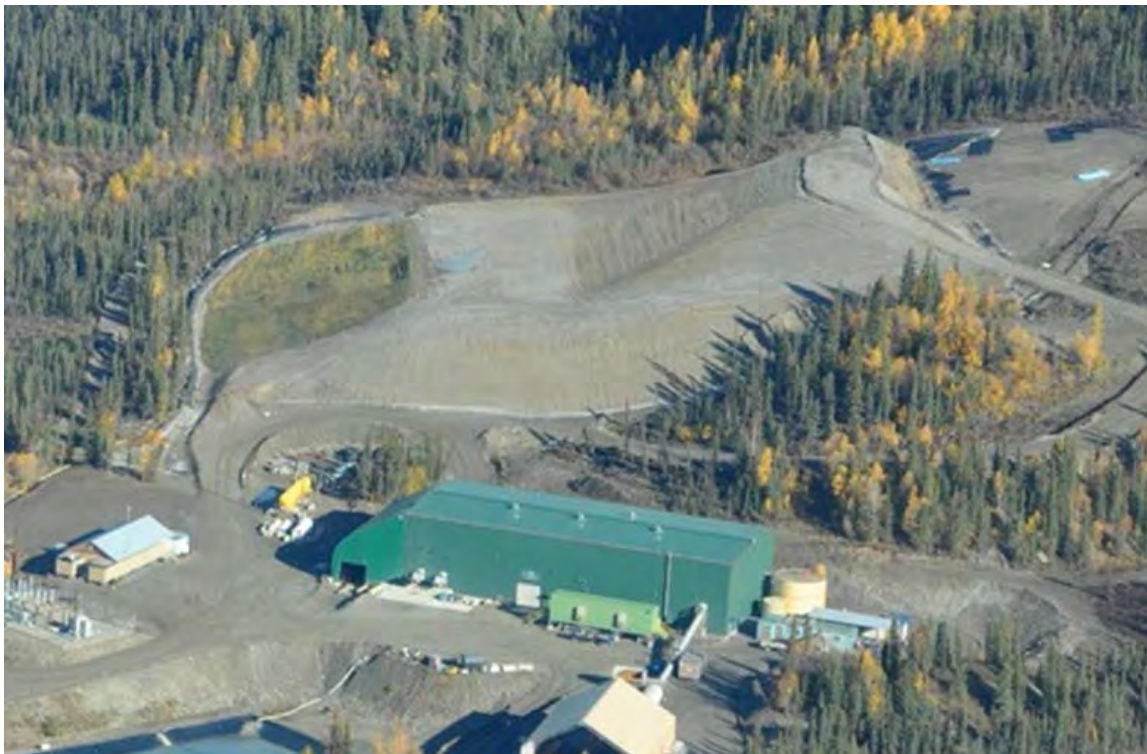
Figure 7-25 DSTF Progressive Reclamation, August 2013
