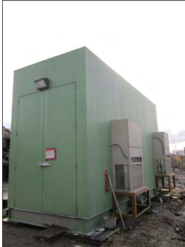
Figure 7-45 Crusher MCC
