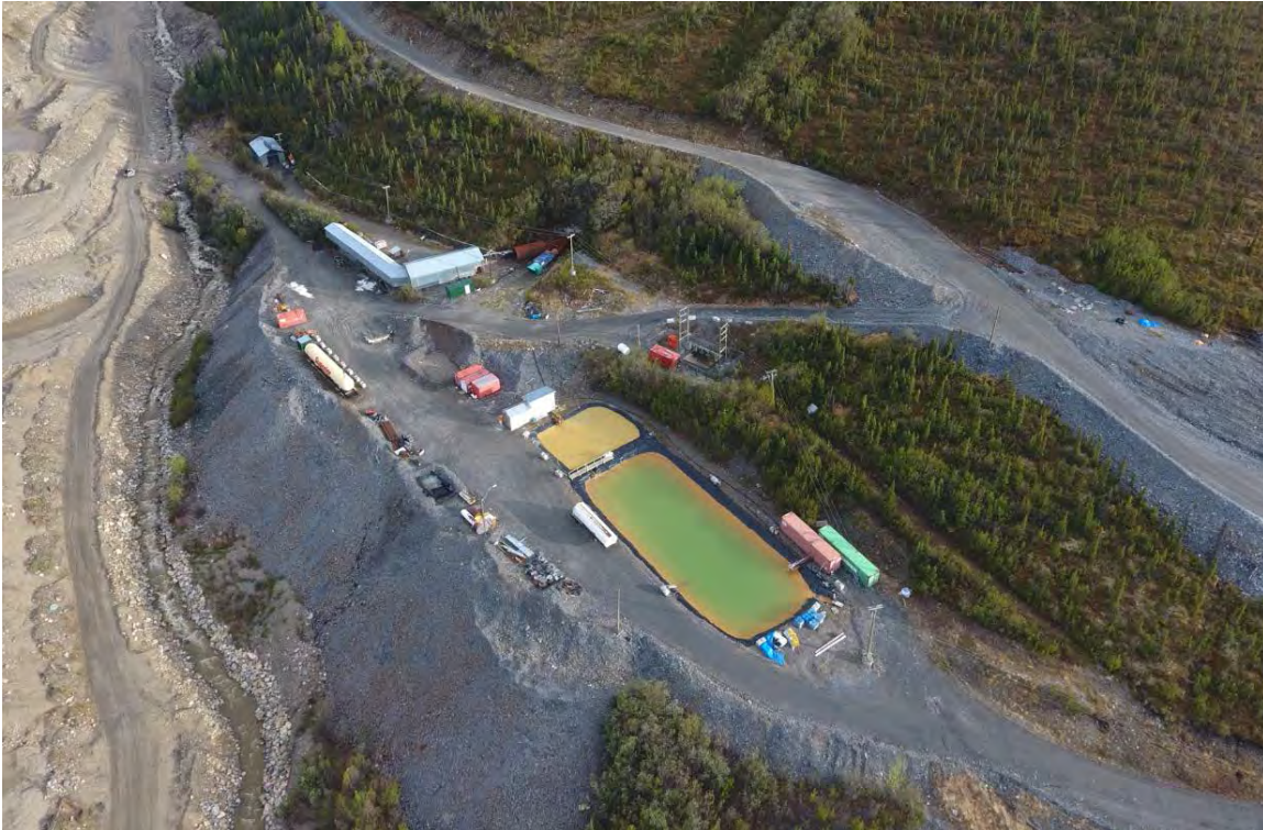
Figure 7-32 Bellekeno 625 WTP Area Overview
