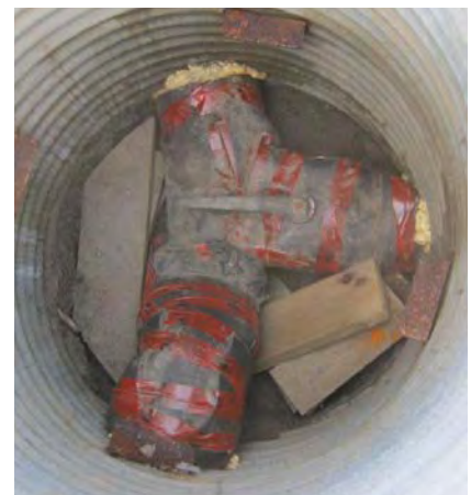
Figure 2 - Inlet Valve
