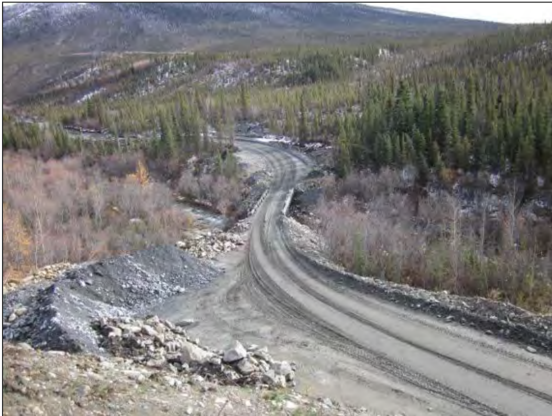
Figure 7-49 Lightning Creek Bridge and Typical Bellekeno Haul Road Section
