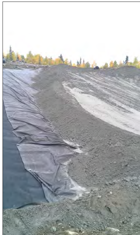
Figure 5-6 Compacted DSTF Lift
