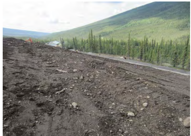
Photo 10: Covered DSTF crest looking south
