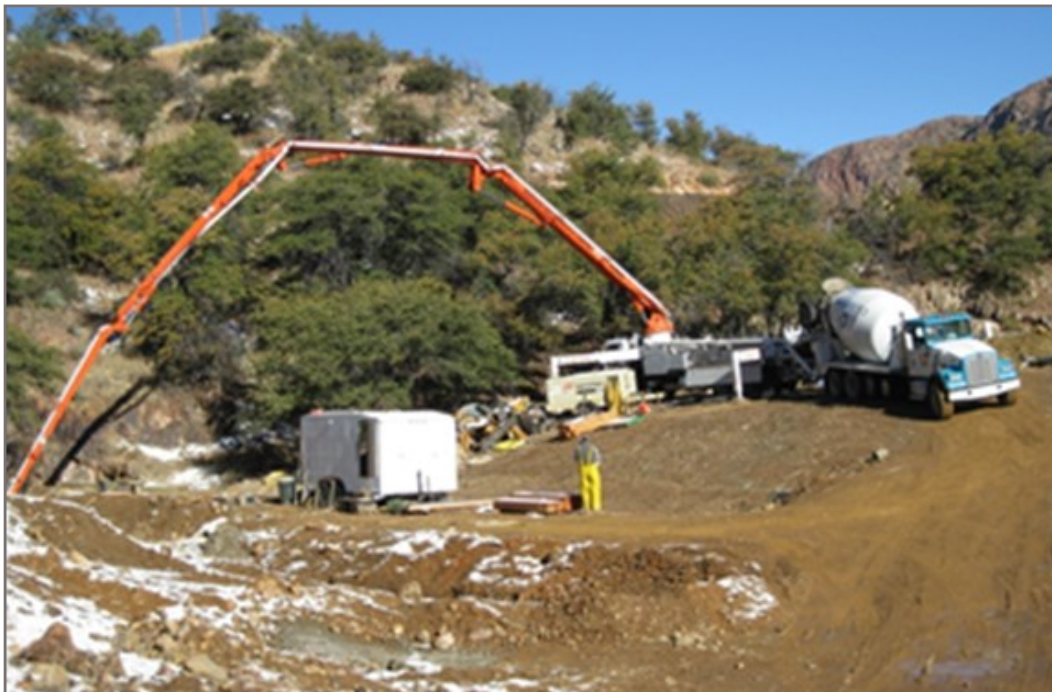
Photo 8: Pumping of grout / cement in several stages
