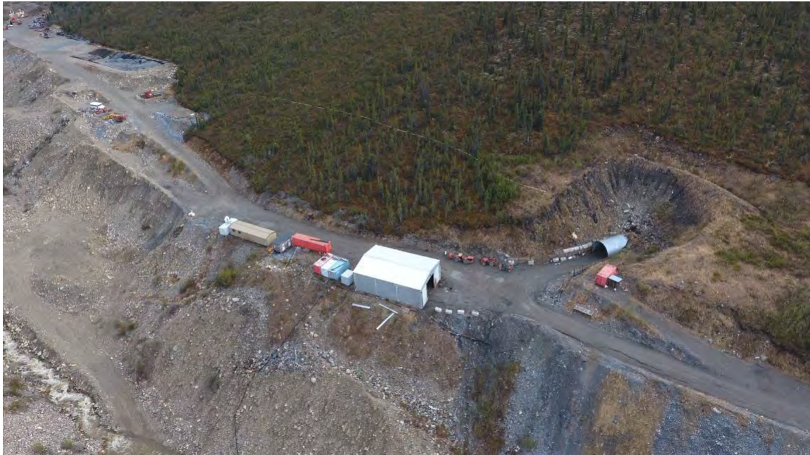
Figure 7-2 Bellekeno East Portal and Site Facilities
