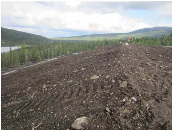
Photo 9: Covered DSTF crest looking north
