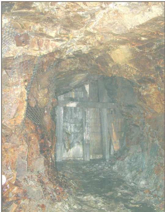
Photo 12: Water tight temporary Bulkhead
