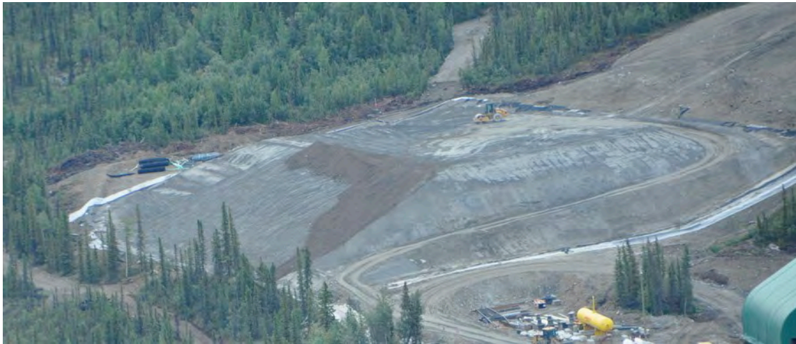
Figure 7-24 DSTF Progressive Reclamation, June 2012
