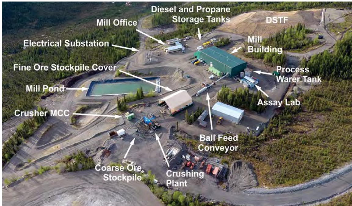
Figure 7-38 Aerial View of Mill Site Infrastructure and Layout
