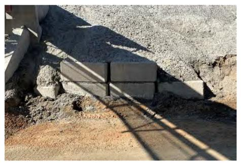
Photo 4: View of mill feed conveyor and bulging lock blocks from the front.
