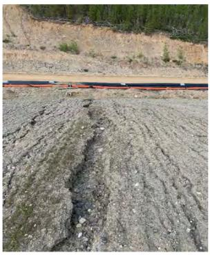
Photo 2: Looking north on MVFE2 at erosion crack (typical).
