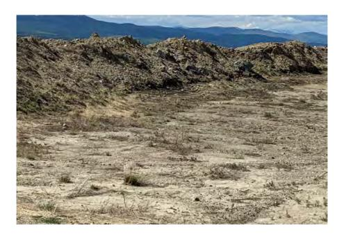
Photo 3: Top of MWD, showing ponded erosion from wave action and high wateer mark.
