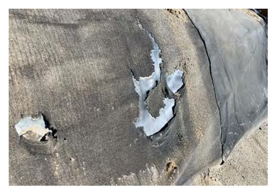
Photo 3: Looking inside containment, bear has damaged filter cloth, but no damage to liner.
