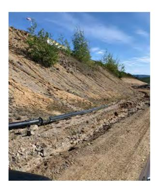
Photo 2: Slope below camp looking east. Note deep erosion channel in road prior to ditch.
