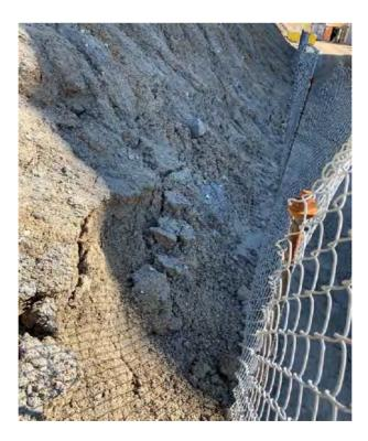
Photo 2: Slope below fuel farm/behind mill looking west. Note undercut slope that needs backfilling.
