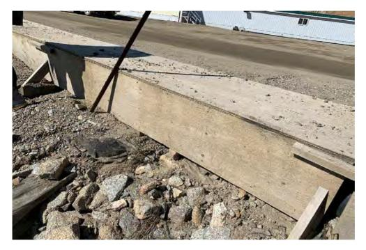
Photo 3: Example of erosion under utilidor.
