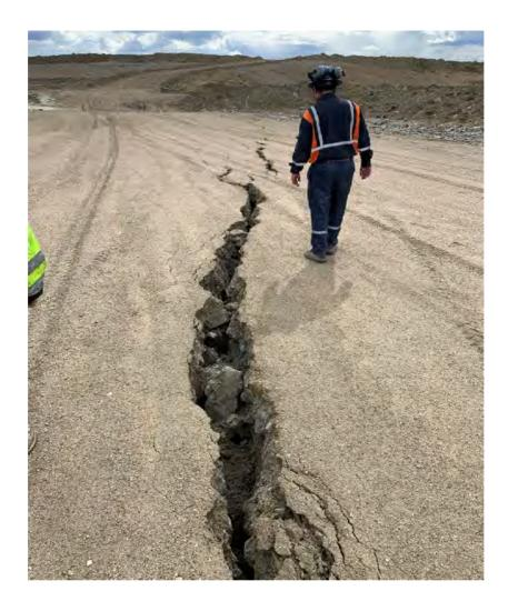
Photo 3: Crack on north side of dump at crest.
