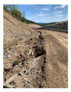
Photo 1: Heavy Erosion channel on North ditch KM 0 - 0.25
