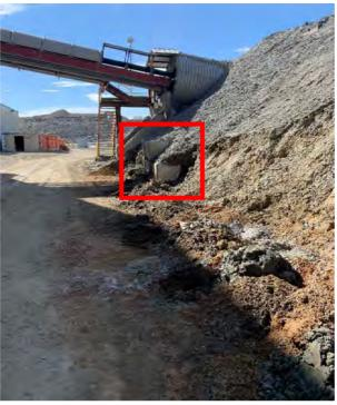
Photo 3: View of mill feed conveyor and bulging lock blocks.
