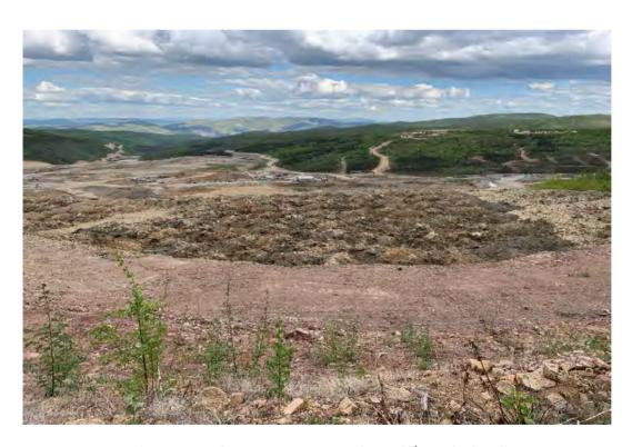
Photo 2: No slumping or issues with north/west highwall.
