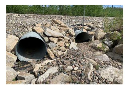
Photo 6: Photo showing gravel movement through culverts
