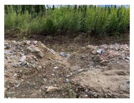
Photo 3: Portion of TDD that appears to have been breached. To be repaired.
