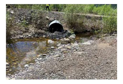
Photo 5: Standing water showing gravel movement through culverts
