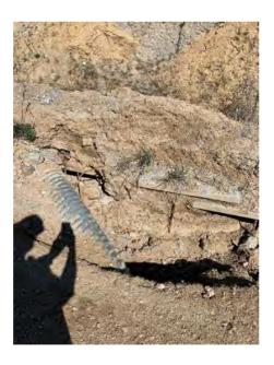
Photo 2: Heavy Erosion channel on North ditch KM 0 - 0.25
