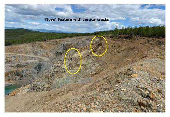
Photo 2: North wall and Vertical Cracks in "Nose" feature
