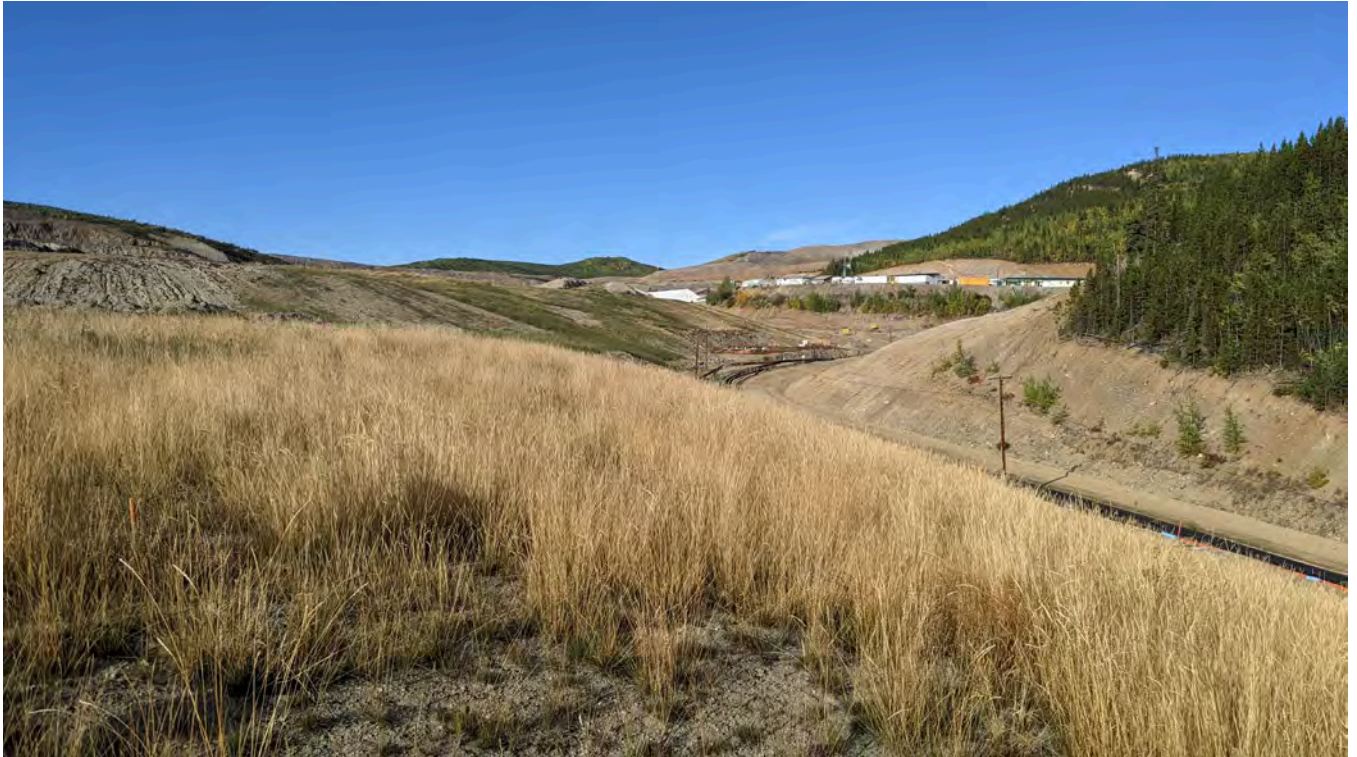
Photo 2-5: View of the north regraded, covered, and vegetated slopes of the MVFE looking towards camp.
