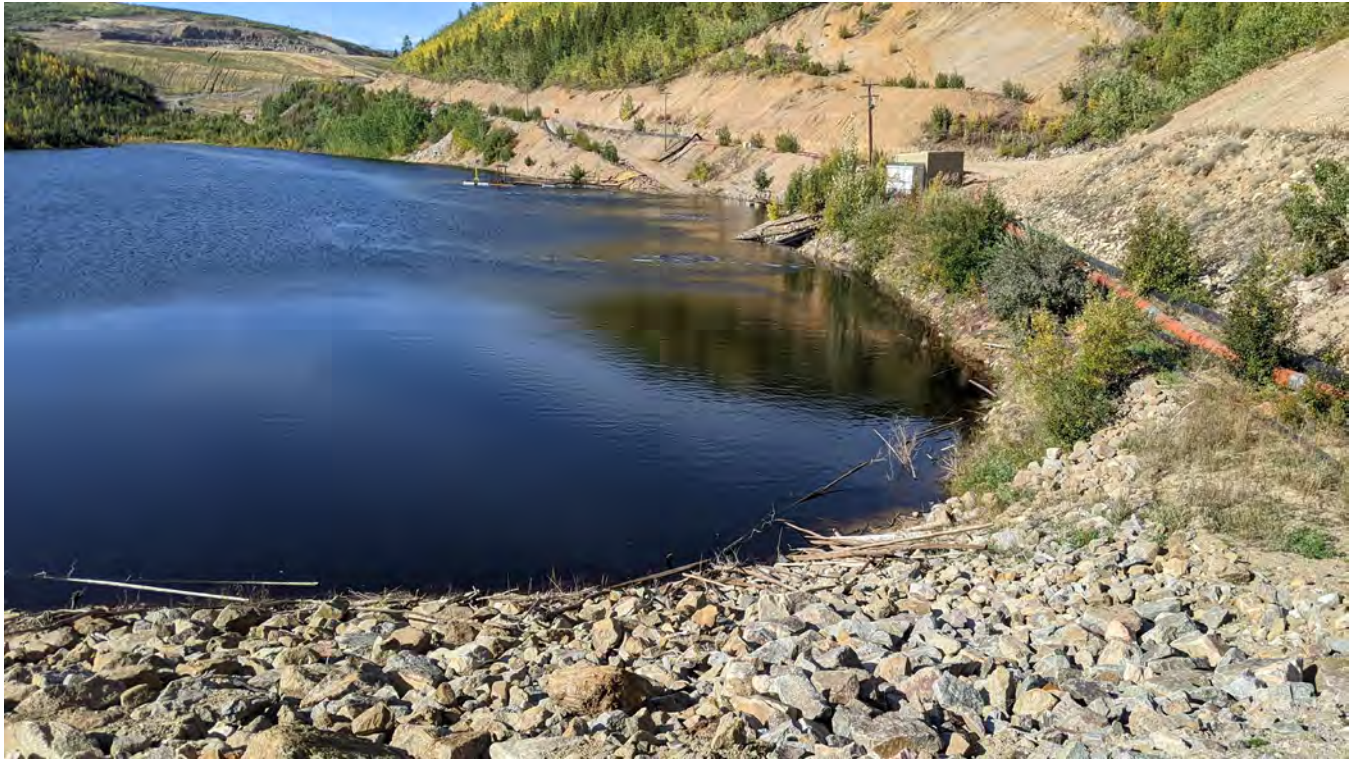
Photo 12-5: Upstream north abutment. The water level in the pond is higher than the previous year, which has resulted in the accumulation of logs across the upstream face of the dam.
