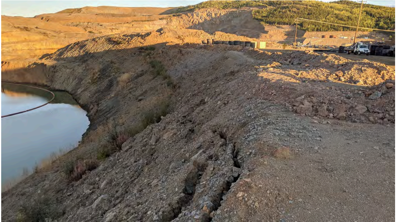
Photo 15-7: Cracking along the Area 2 Stage 3 Pit rim.
