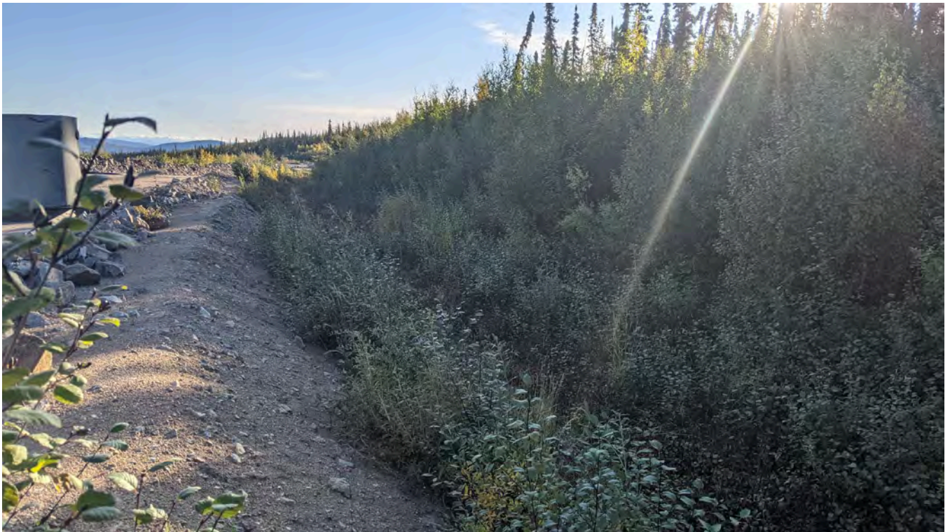
Photo 3-4: Vegetation in the upper portion of the TDD looking downstream.
