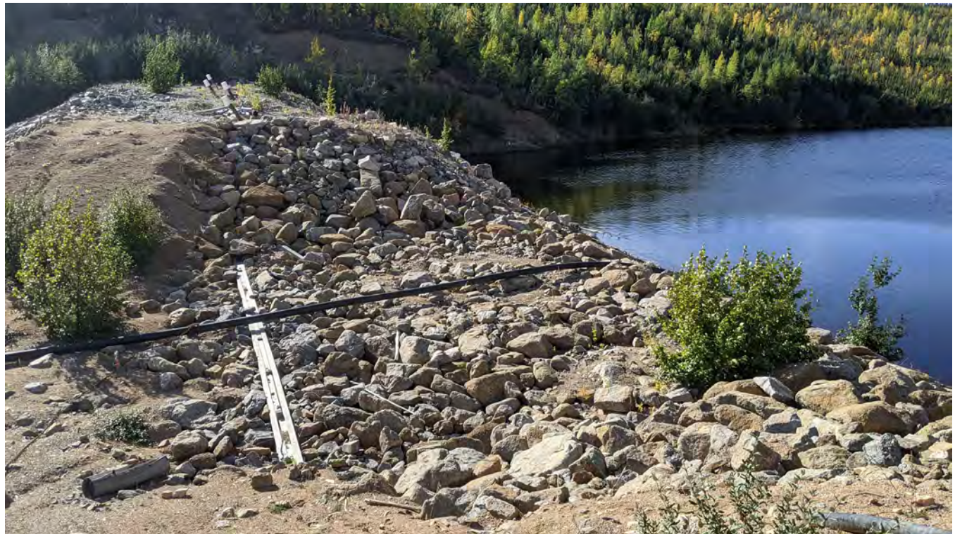
Photo 12-4: WSP spillway looking south from the dam crest.
