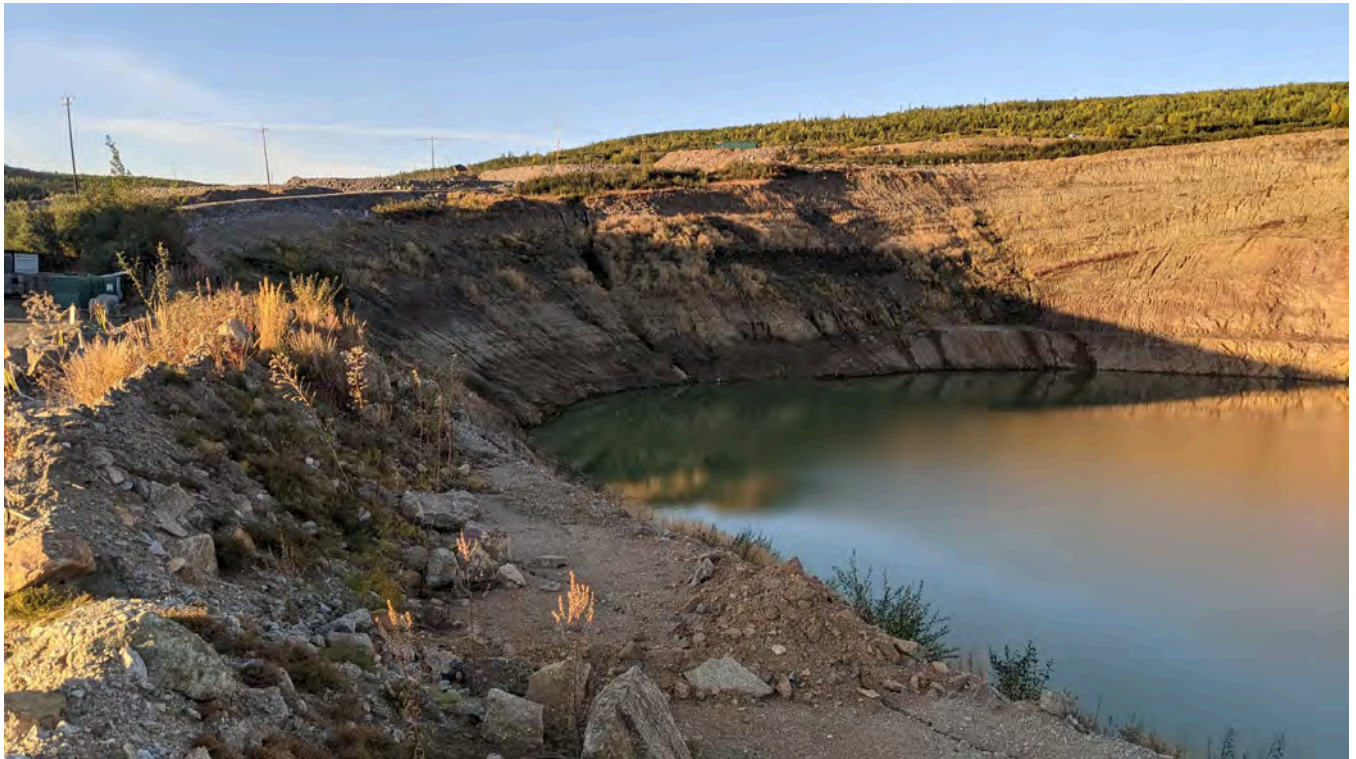
Photo 15-6: Area 2 Stage 3 Pit looking south.
