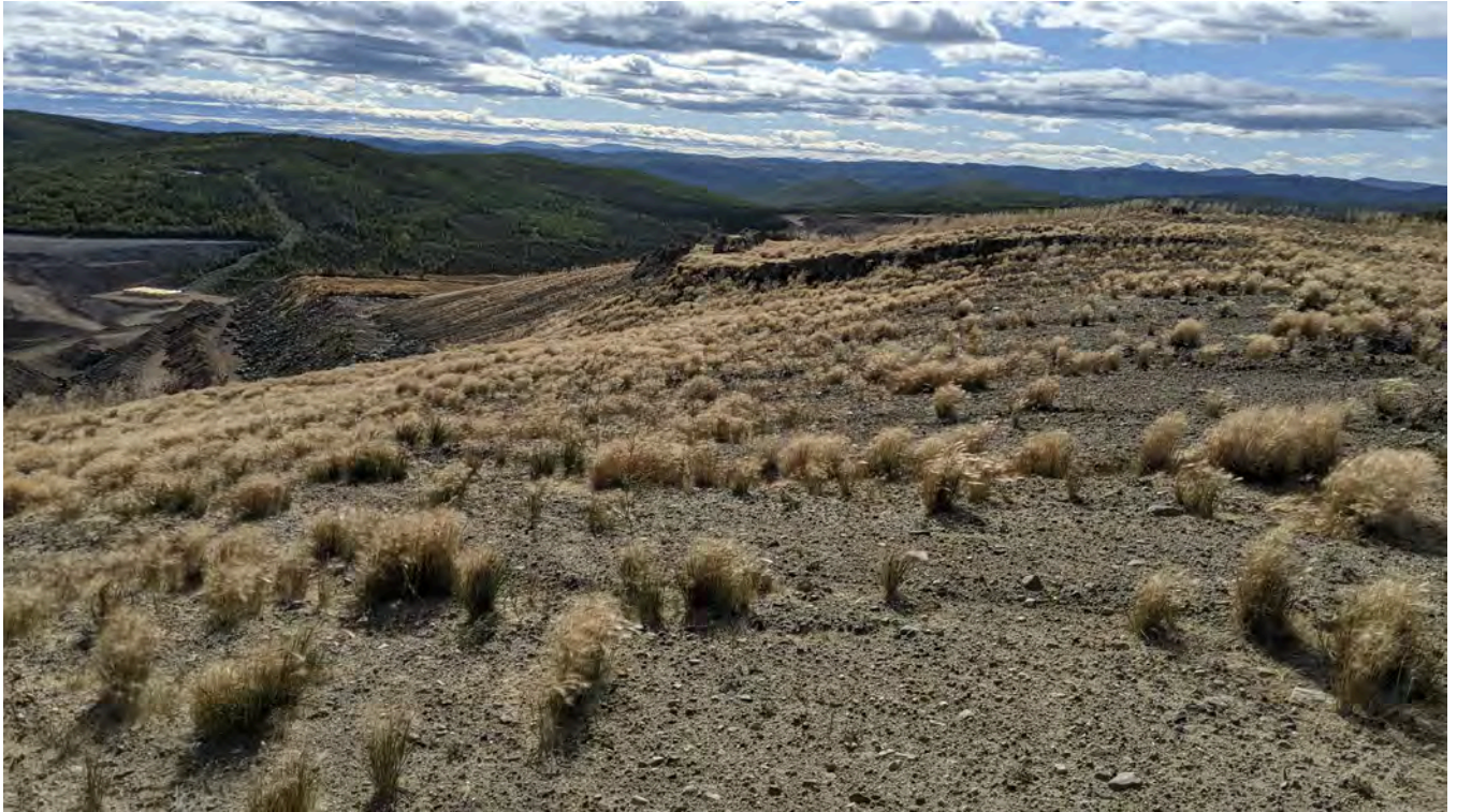
Photo 4-1: MWD regraded slope (looking southeast). A stockpile of cover soil is visible that is located above a portion of the dump that remains to be regraded.
