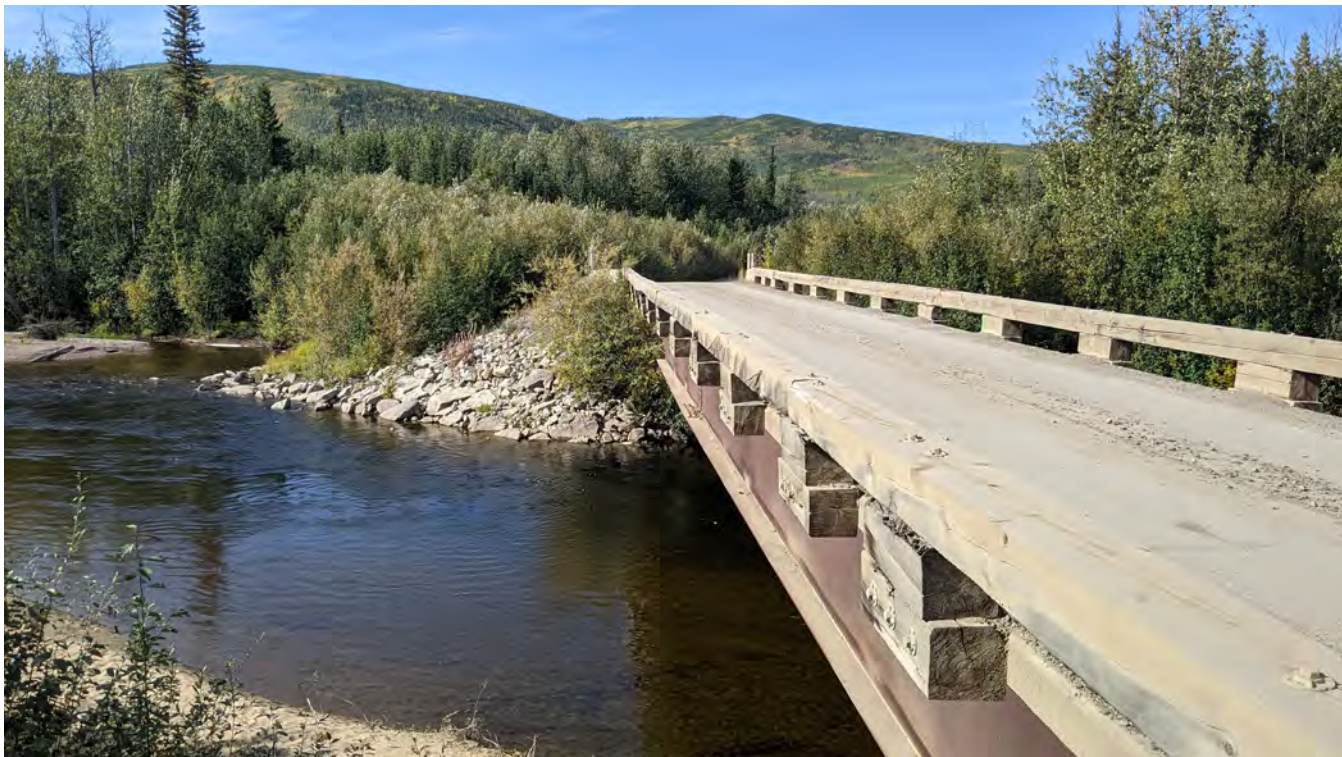
Photo 13-1: Western bridge abutment.
