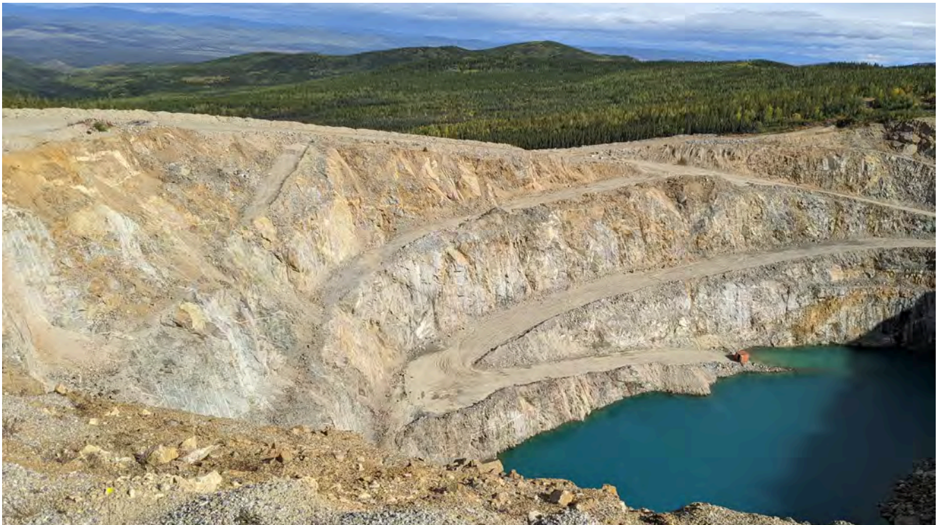
Photo 17-2: North pit wall.
