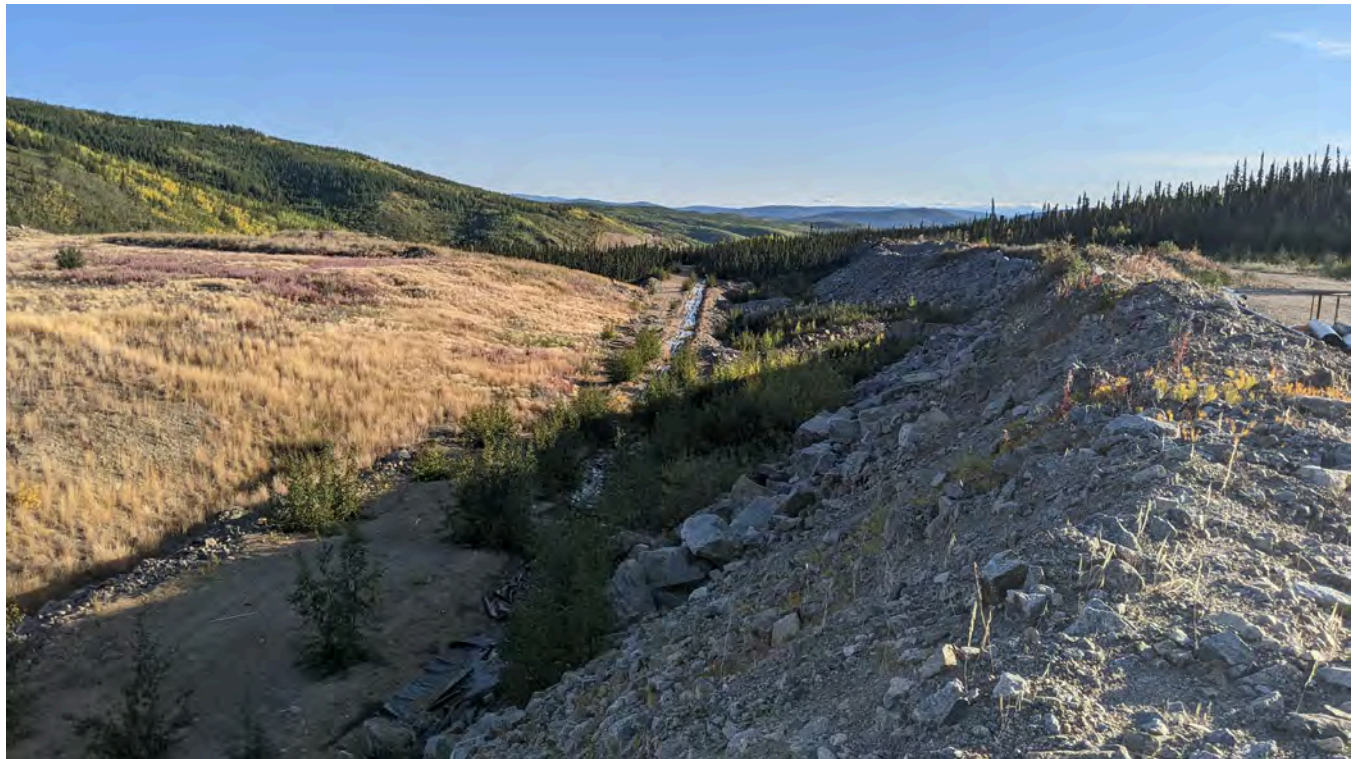
Photo 1-2: Southeast end of the DSTSF from TDD road (looking east)
