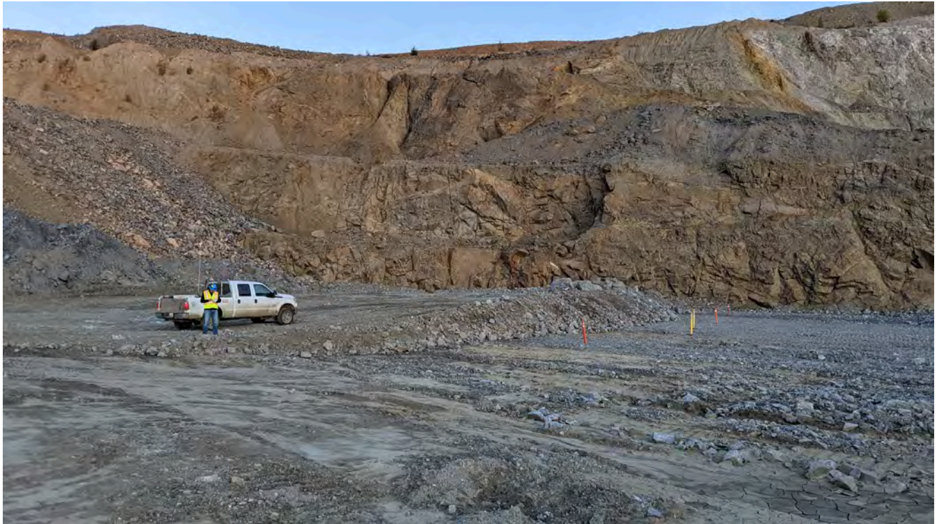
Photo 14-7: SAT Dump. An additional lift of SAT material has been placed on the SAT Dump in the past year. If the Main Dam does not proceed, this additional material will need to be relocated below the long-term water level.
