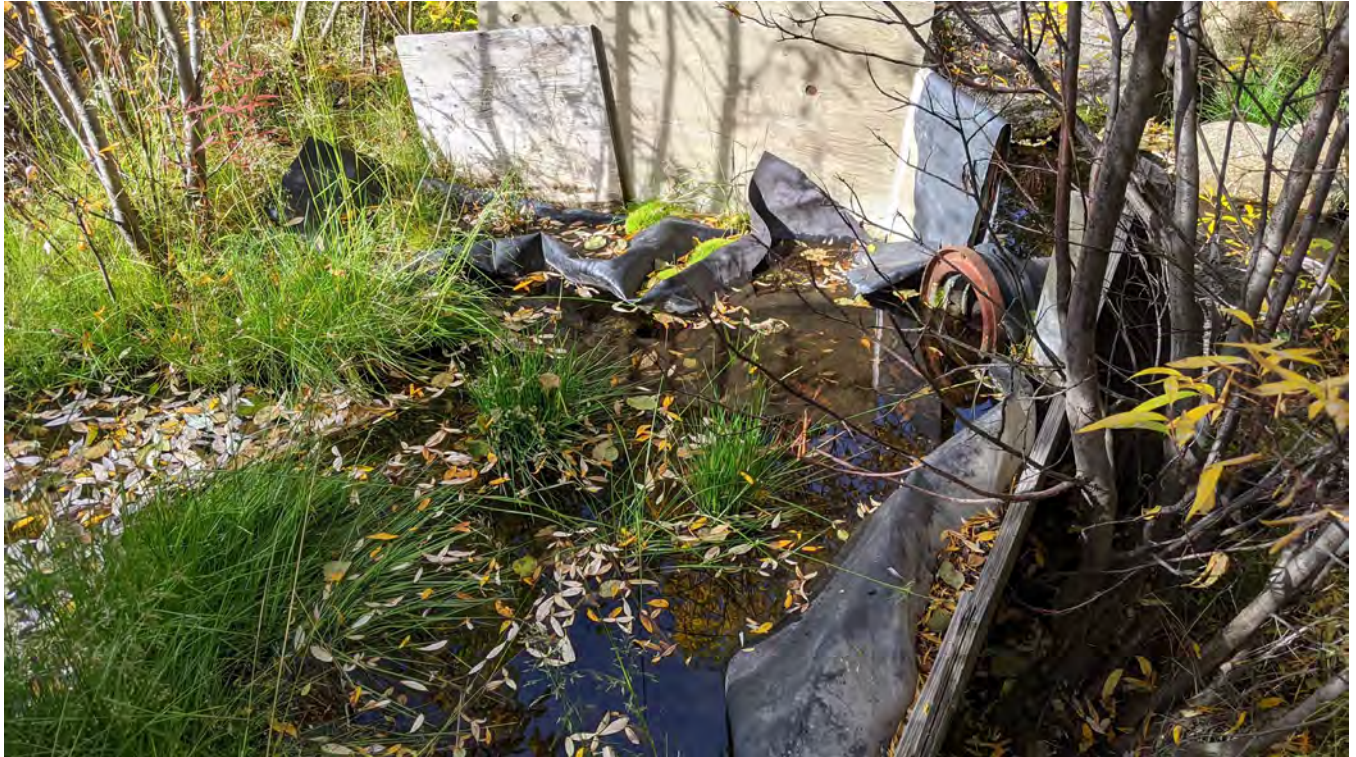
Photo 12-9: View of the seepage weir downstream of the dam.
