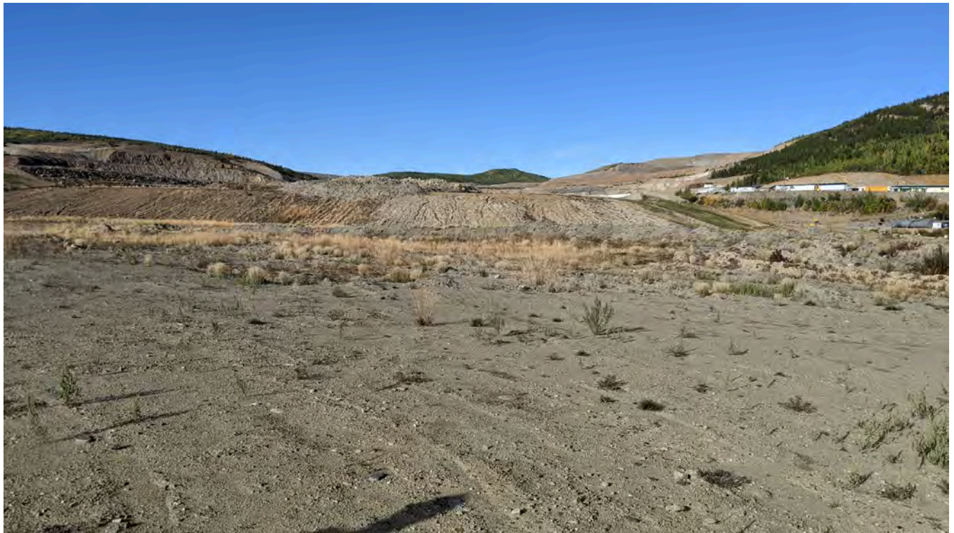
Photo 2-2: Looking west across Tier C, minor erosion gullies visible down Tier B of the MVFE.
