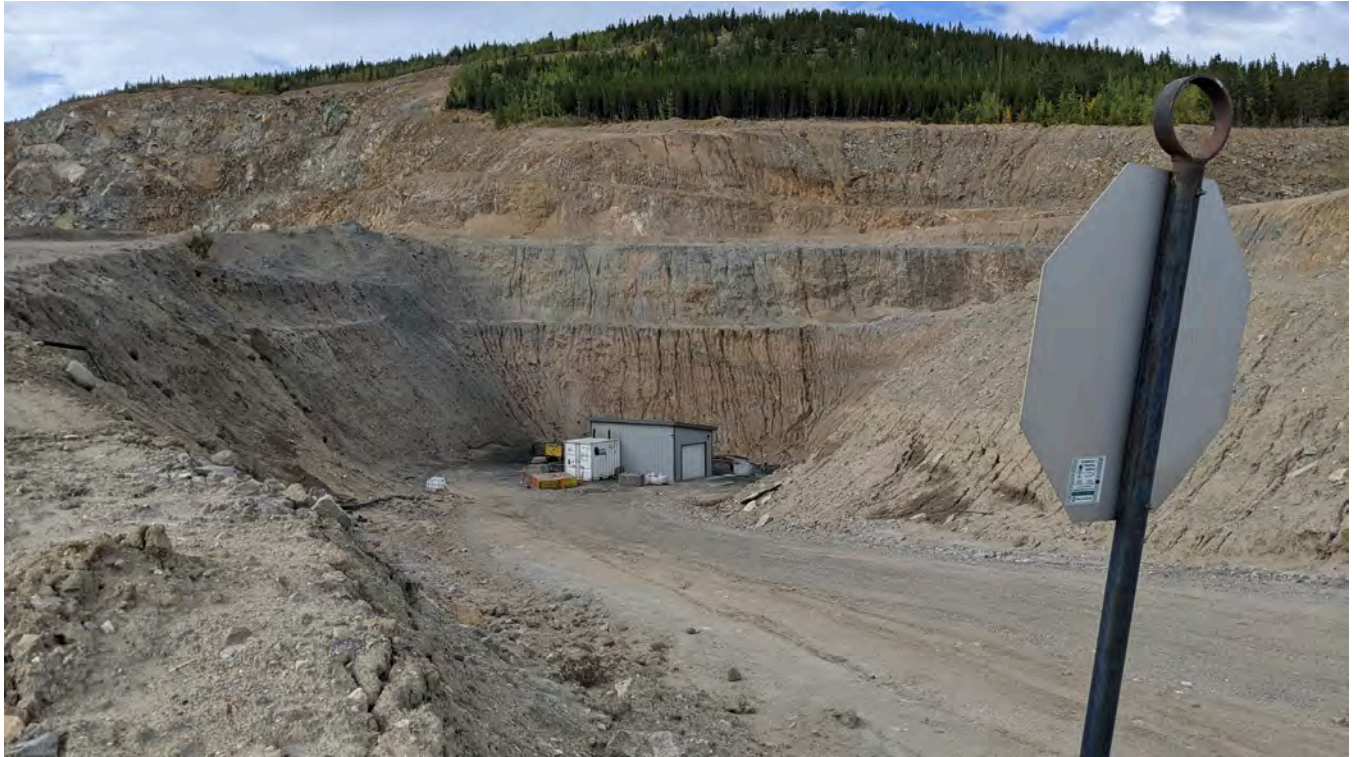
Photo 14-5: Vent raise located west of the Main Pit.
