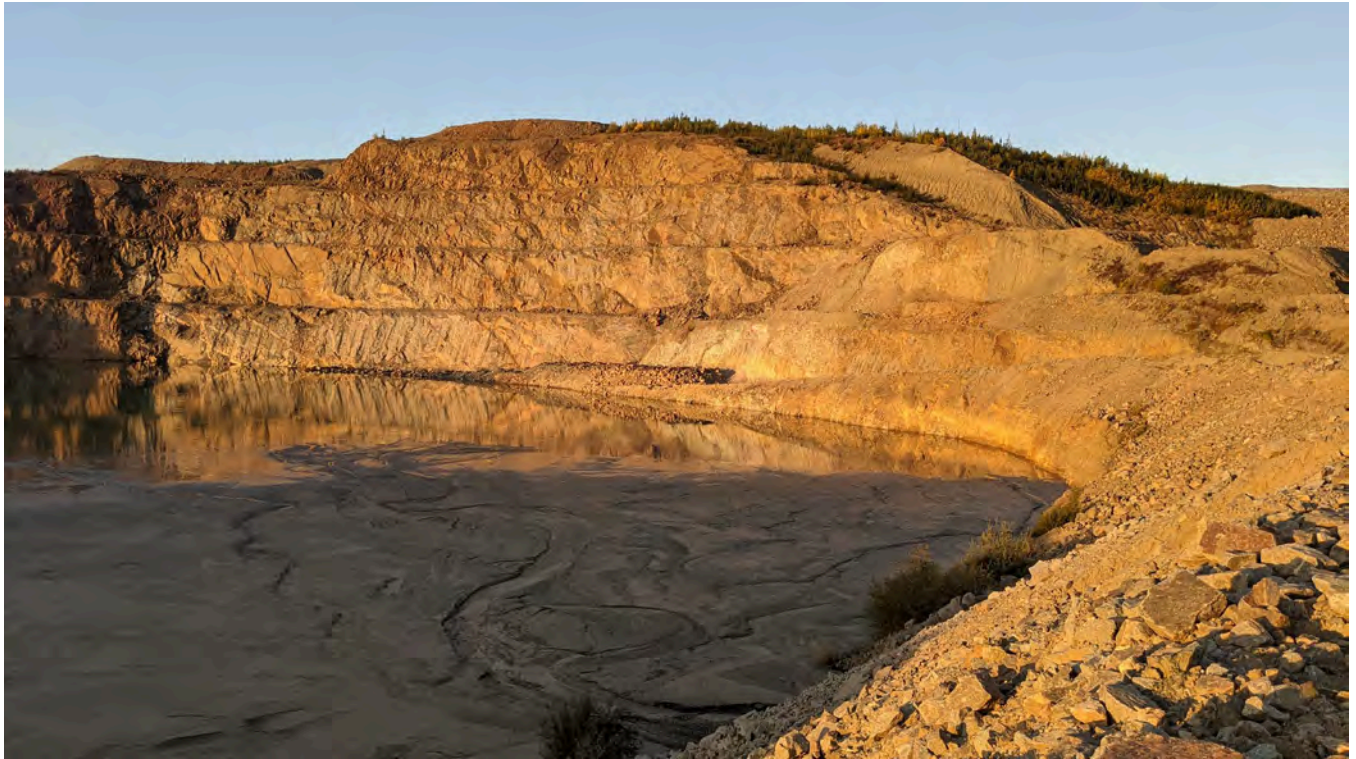
Photo 15-1: Area 2 Stage 2 Pit backfilled with tailings looking southwest
