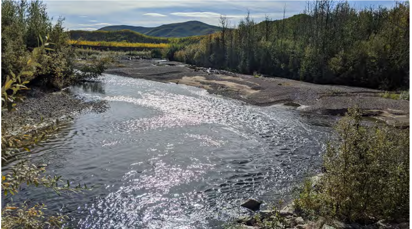
Photo 13-3: Big Creek looking upstream from the western abutment. An eddy is present upstream of the west abutment. The condition of the eddy and creek is the same as the 2020 inspection.
