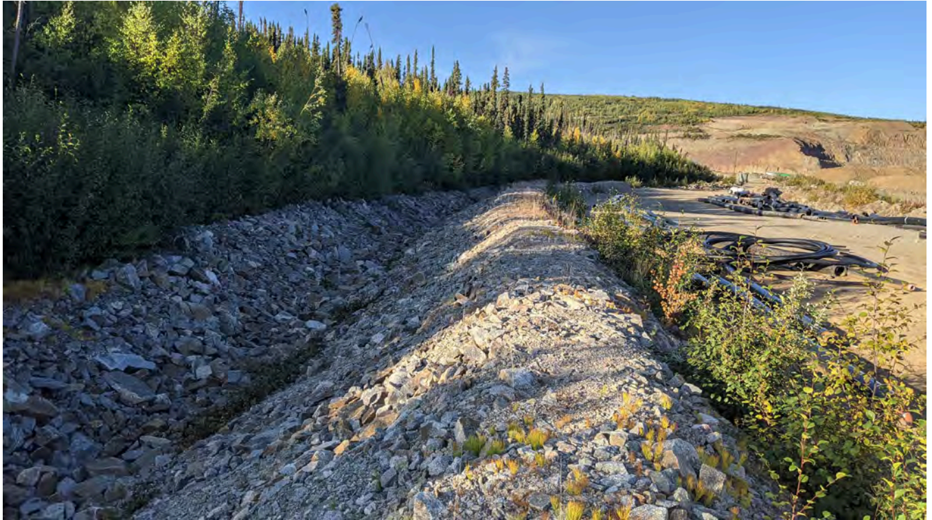
Photo 3-5: Typical view of the lower portion of the TDD with riprap. Sparse vegetation growing in the channel.
