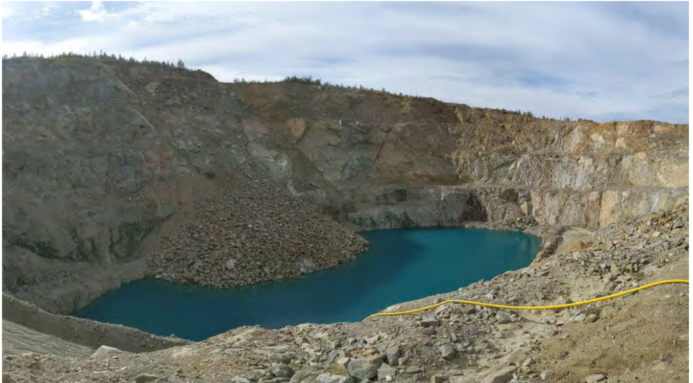
Photo 17-1: Previous pit wall failure in Minto North Pit (looking southwest).
