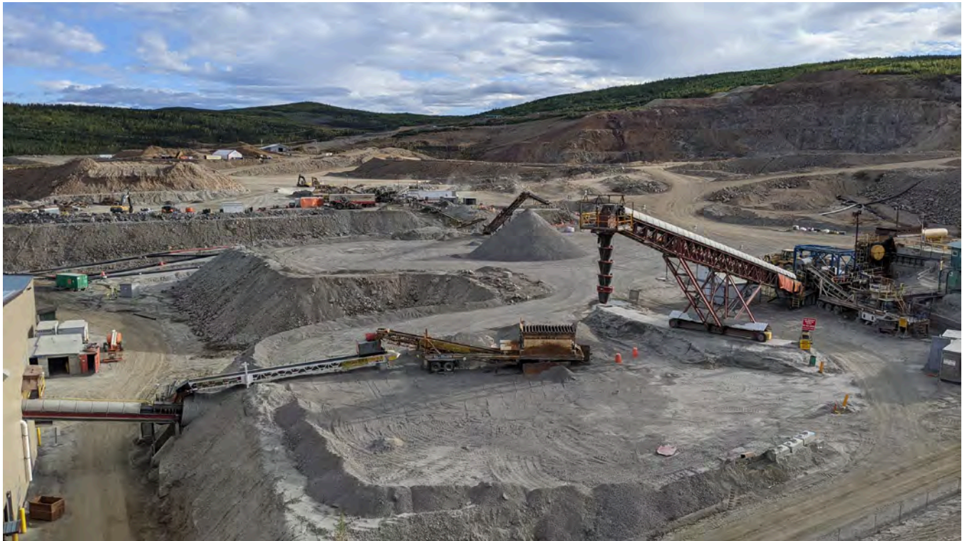
Photo 8-1: Crusher Stockpile west of the mill.
