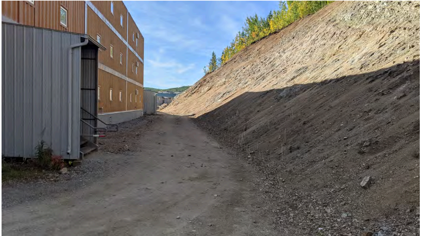
Photo 10-1: Highwall behind Selkirk Manor looking south from the north end of camp.
