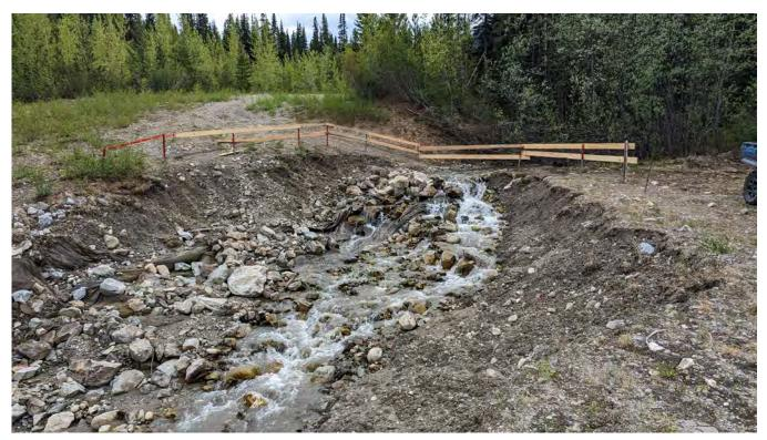
Photo NC-06: On-going erosion at the North Creek second crossing (to landfill) looking upstream.
