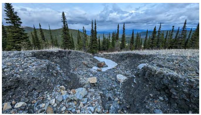
Photo WR-04: Erosion at the lowest point of the Jewelbox Waste Rock Dumps through the former Jewelbox Haul Road (looking north). Erosion has developed down to bedrock. Extent of erosion is unchanged compared to 2022 inspection.
