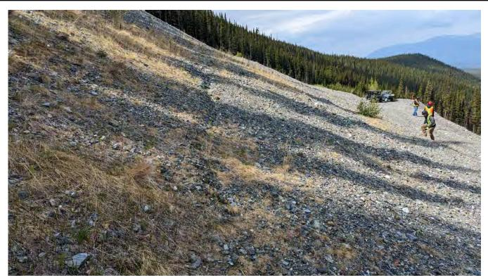
Photo WR-11: Regraded Burnick Waste Dump at the 1200 Portal. A crack is present above the portal that is approximately 10 m long, up to 15 cm wide, and up to 10 cm deep.
