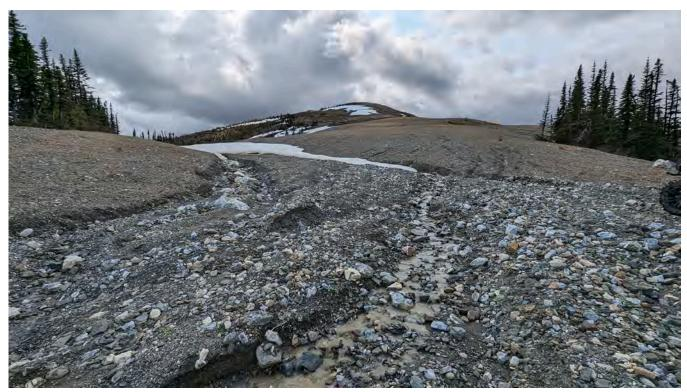
Photo WR-03: Erosion at the lowest point of the Jewelbox Waste Rock Dumps through the former Jewelbox Haul Road (looking south).
