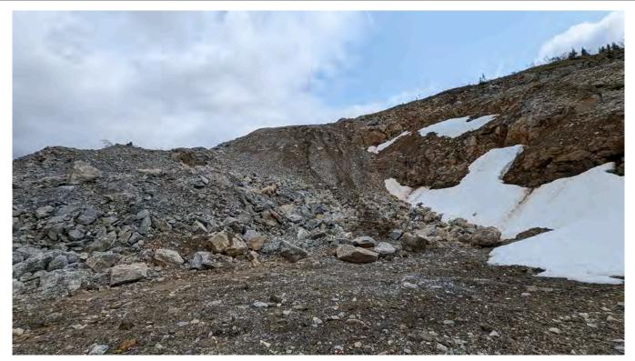
Photo WR-09: Backfill at the 1380 Portal below the Main Zone Waste Rock Dump.
