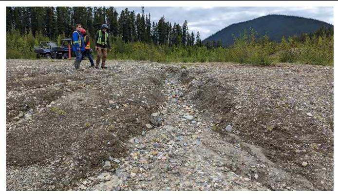
Photo L-3: Erosion channel that enters the Landfill drainage channel. The condition of the channel is unchanged compared to the 2022 inspection and no signs of debris were observed.
