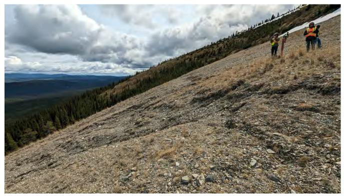
Photo WR-05: Surficial slumping near the south end of the 1408 Portal Waste Rock Dump.
