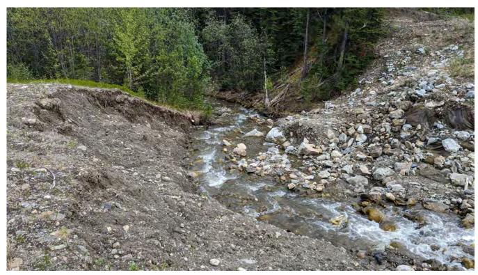
Photo NC-05: On-going erosion at the North Creek second crossing (to landfill) looking downstream.
