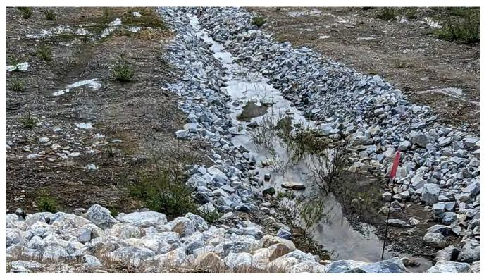
Photo DC-01: Upstream end of the South Drainage Channel immediately downstream of the SRS Spillway. Sediments are accumulating in the channel due to erosion at the base of the SRS spillway.
