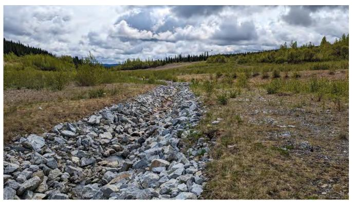
Photo DC-02: Downstream end of the South Drainage Channel looking downstream towards the confluence with the Camp Creek Channel Iron-staining on the riprap is present over the last 30 m of the channel.
