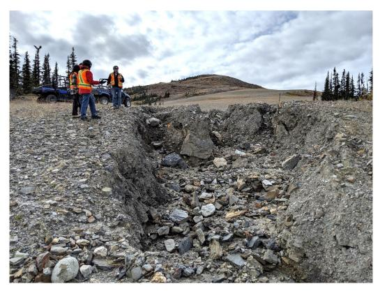
Photo 25: Erosion gully at toe of Jewelbox Waste rock dump
