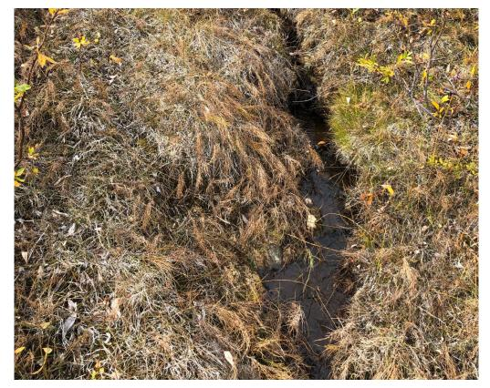
Photo 6: Seepage at toe of North Dam, mainly due to hillside springs
