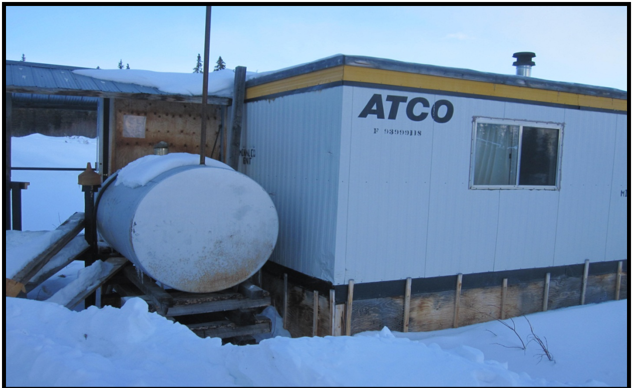
Photo 2-3: Diesel tank for heating fuel with about 1000 litre capacity (photo: March 19, 2011)
