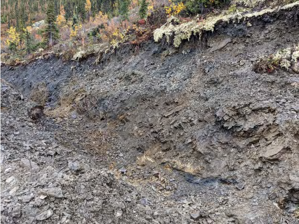
Figure 10: Trench BHU3 in use
