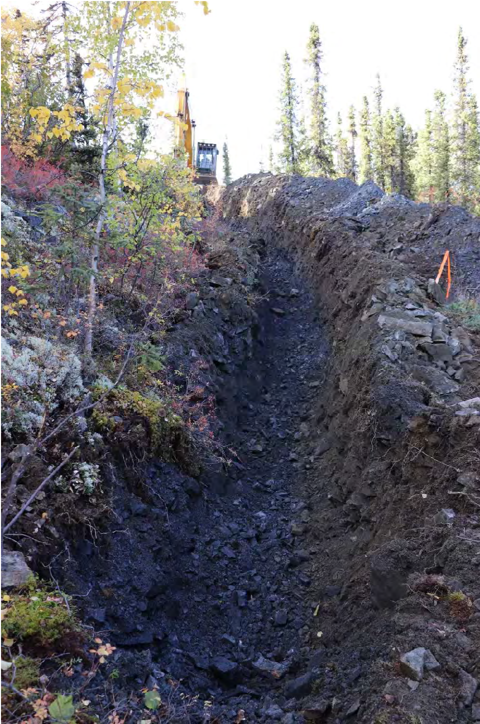
Figure 5: Trench BHU2 while active.
