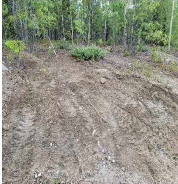
A disturbance (08 V 611342, 6881611) was back filled with adjacent material and then seeded.
