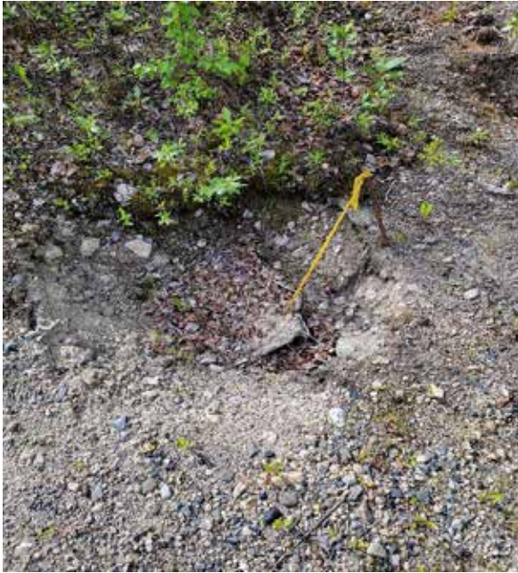
Collapsed drill hole (08 V 611272, 6881612)
