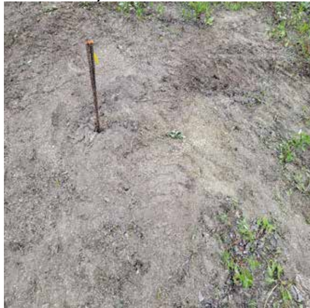
The drill hole was backfilled and seeded. The rebar that was found in the hole was placed back on the drill hole.
