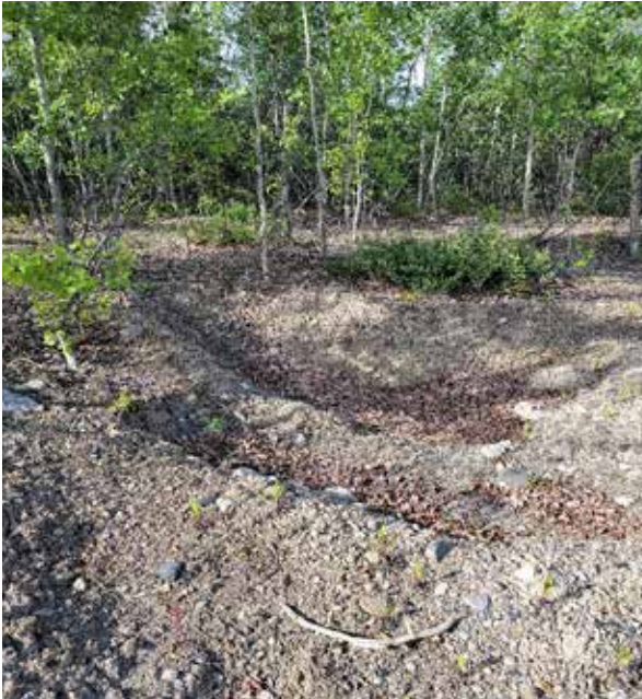
A disturbance (08 V 611342, 6881611) was back filled with adjacent material and then seeded.
