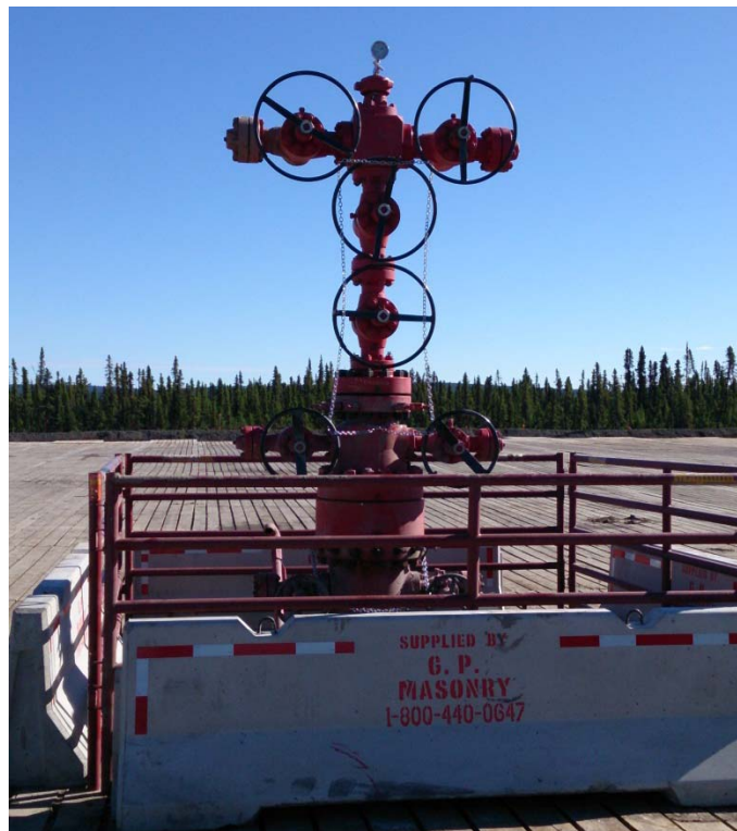
Figure 3: B-73 Wellhead Final Installation
